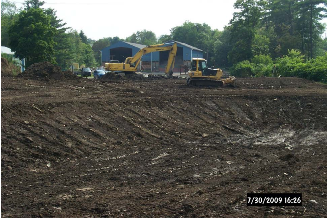
Construction of the settling pond/wetland downstream of the AFVFP.
