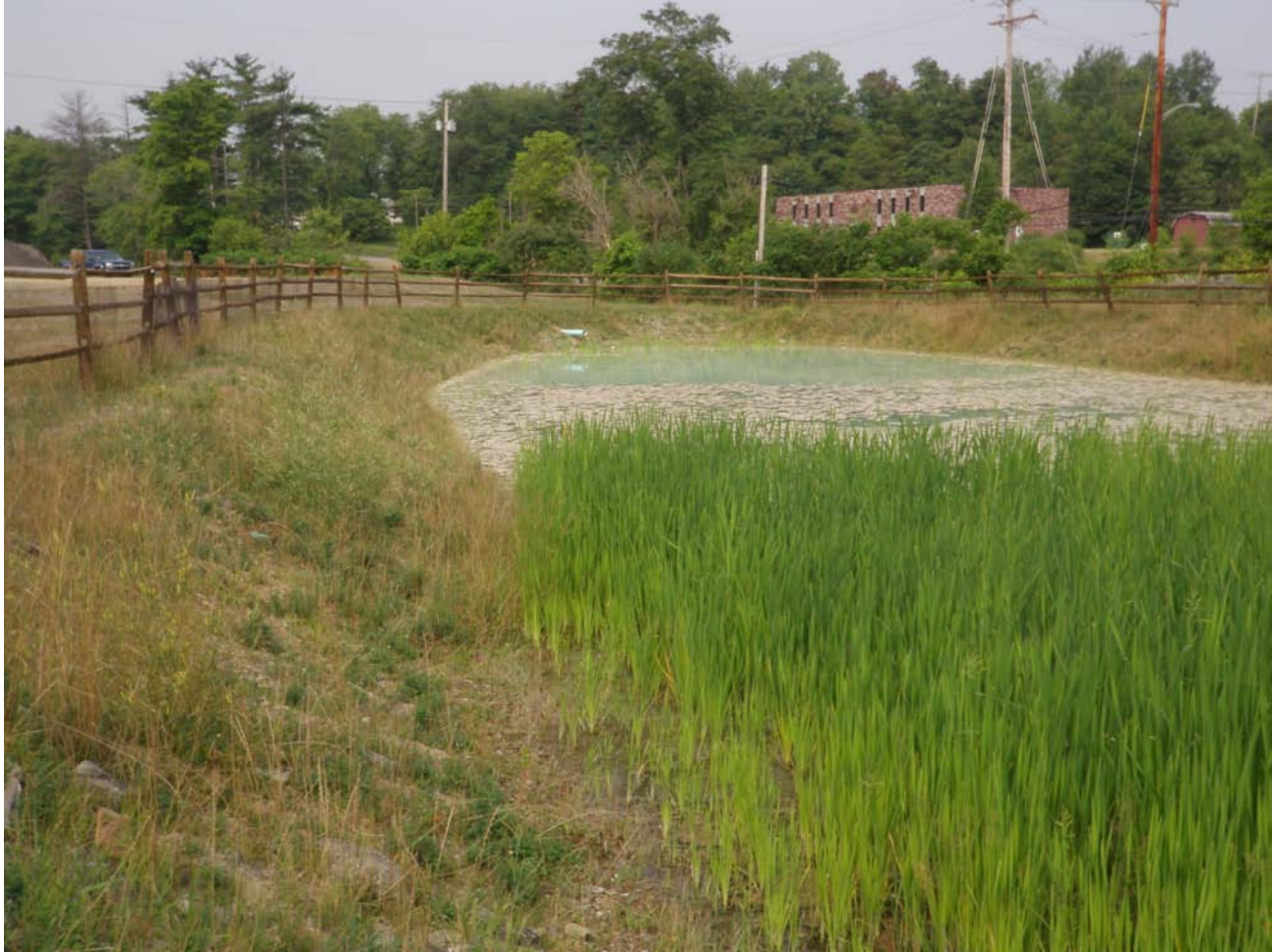
View of Settling Pond (back ground) and Wetland (foreground) with safety fence.
