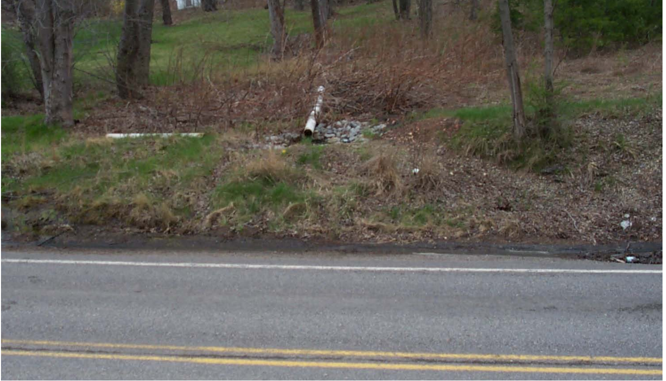
MP5 discharge prior to treatment issuing from existing 6" PVC pipe flowing into storm water facilities along Clinton Road (SR-3089).
