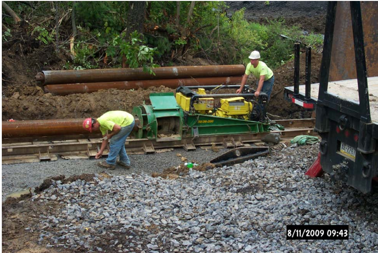
Centerline Boring, Inc. of Zelienople, PA installing 12" diameter steel casing. The horizontal bore crossed under an 8" water line owned by Findlay Township Municipal Authority, Clinton Road (SR3089), and a 4" steel Dominion Peoples gas line
