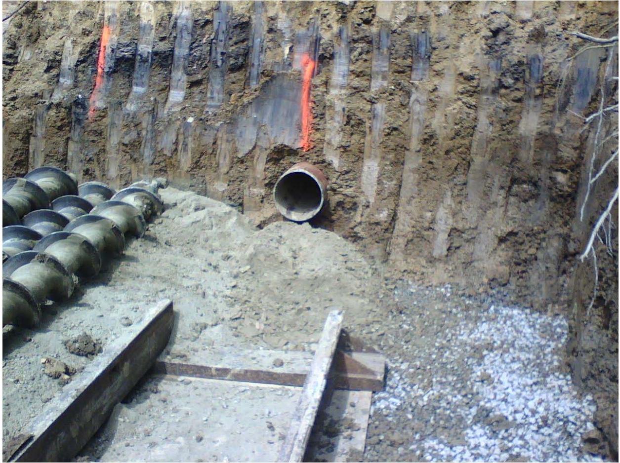
80' long 12" diameter steel casing installed beneath Clinton Road to conduct the AMD discharge to the treatment facility. A six-inch SCH40 PVC pipe was inserted into the steel casing.
