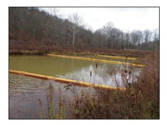
The Kolb Passive Treatment System has a fountain (*left*) to help aerate the net-alkaline, iron-bearing discharge. Additional baffle curtains (*right*) were purchased through the O&M grant and installed by the BCWA to help improve retention and iron removal.
