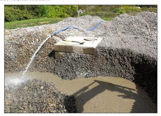
Poor effluent quality at the McCaslin Road PTS indicated the need for maintenance. In September 2012, the aluminum- and iron-coated limestone aggregate *(bottom)* in the Auto-flushing Limestone-only Vertical Flow Pond was cleaned using a small excavator to handle and to stir the limestone aggregate while using a pump to wash off the coating *(top)*. The sludge material that was removed from the limestone aggregate was then flushed into the settling pond.
