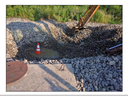
**Above:** The aluminum and iron-coated limestone aggregate in the Auto-flushing Limestone-only Vertical Flow Pond was cleaned.
