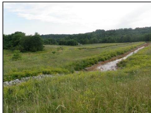
The most recent restoration efforts included the recovery of 37,608 tons of acid-producing coal refuse for power generation and the construction of three oxidation and precipitation channels (**OPCs**)
