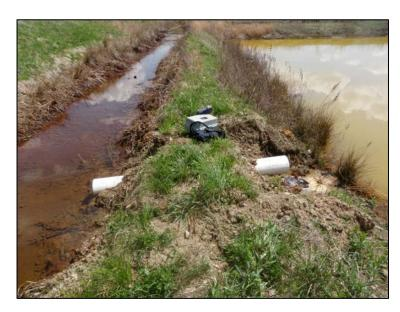
**Top Left:** Forebay effluent pipes extended into the middle of the Forebay which would plug with low pH iron and frequently need to be cleaned.
