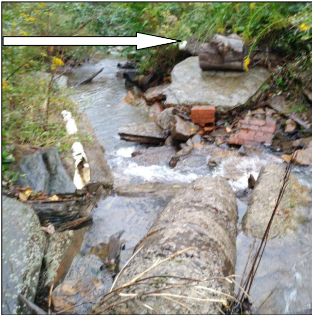
Top Left: Lower system discharge collection and conveyance pipe from mine seal has been damaged. Top Right: Pieces of the broken collection system conveyance pipe were still present in the stream channel. Bottom Left: Water was poured into the damaged pipe to confirm it flowed to the system. Bottom Right: Upper System VFP no longer appeared to be passing water through the media.
