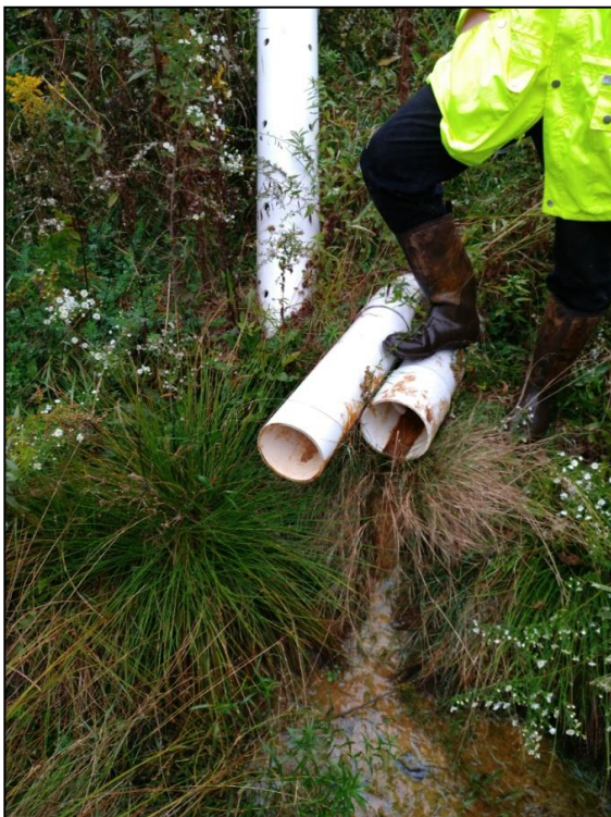
Top Left: Lower system discharge collection and conveyance pipe from mine seal has been damaged. Top Right: Pieces of the broken collection system conveyance pipe were still present in the stream channel. Bottom Left: Water was poured into the damaged pipe to confirm it flowed to the system. Bottom Right: Upper System VFP no longer appeared to be passing water through the media.
