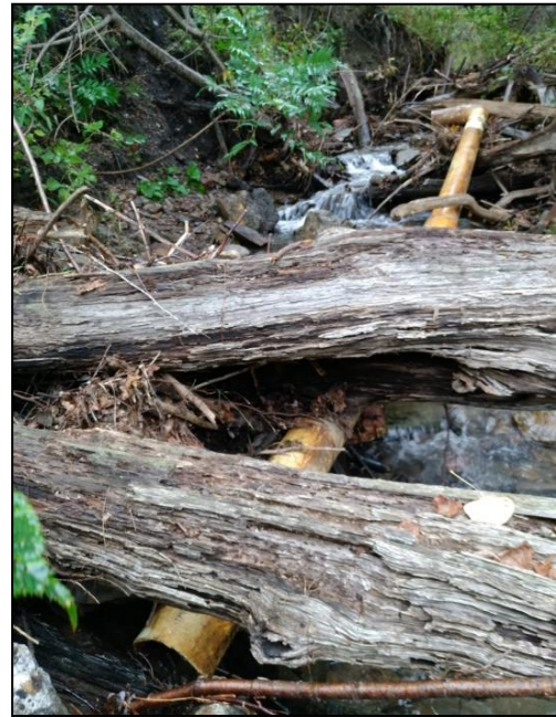
Top Left: Lower system discharge collection and conveyance pipe from mine seal has been damaged. Top Right: Pieces of the broken collection system conveyance pipe were still present in the stream channel. Bottom Left: Water was poured into the damaged pipe to confirm it flowed to the system. Bottom Right: Upper System VFP no longer appeared to be passing water through the media.
