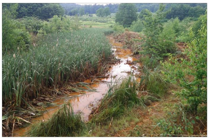
**Top Left:** Water was short circuiting and exiting the emergency spillway due to a buildup of vegetation. **Top Right:** The spillway between the settling pond and polishing wetland was cleared of vegetation, allowing flow to remain in the system.
