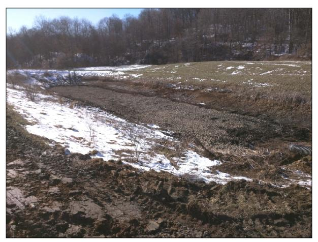
**Top Left:** VK2 was drained revealing 6-8" of sediment on top of the limestone which was removed.
