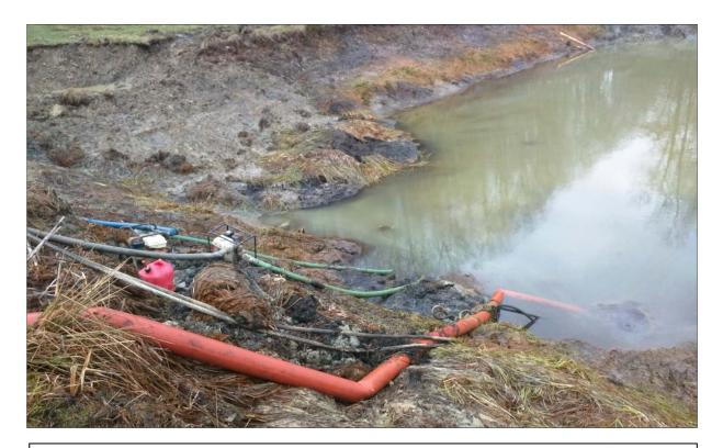
**Above:** As the underdrain was not functioning, VK1 was pumped to gain access to the media.
