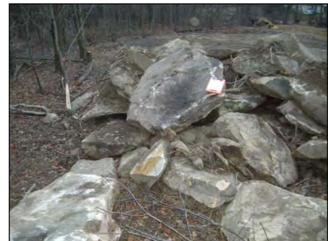
Once the passive system design and associated permitting were completed, the construction area was cleared and grubbed (Top Left and Right). Next, earth material was excavated using a dozer and excavator to the design elevation of the system. Suitable material from the excavation was used to construct the embankments for the passive system. Large boulders encountered during construction were placed to provide wildlife habitat (Bottom Right).
