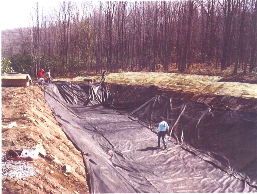
Placing Geotextile Liners – April 2006
