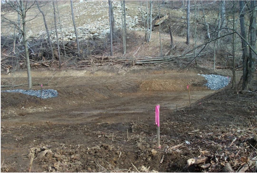
Picture 3: Construction of treatment cell 1
