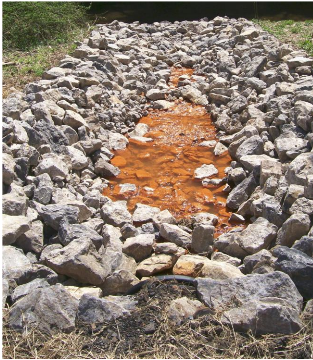
Picture 14: Detail of discharge channel to Carnahan Run
