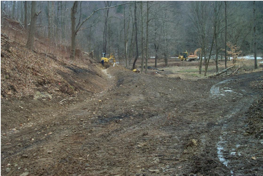
Picture 2: Construction of delivery channel
