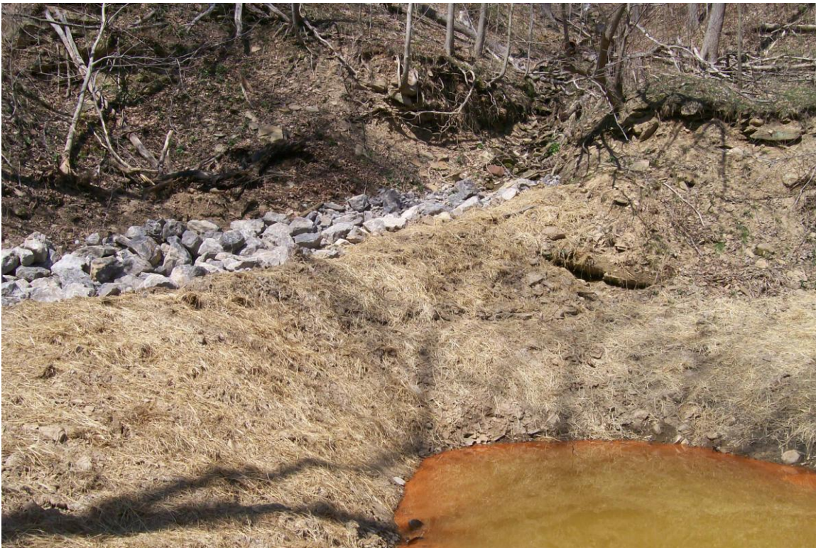
Picture 8: Surface water diversion channel
