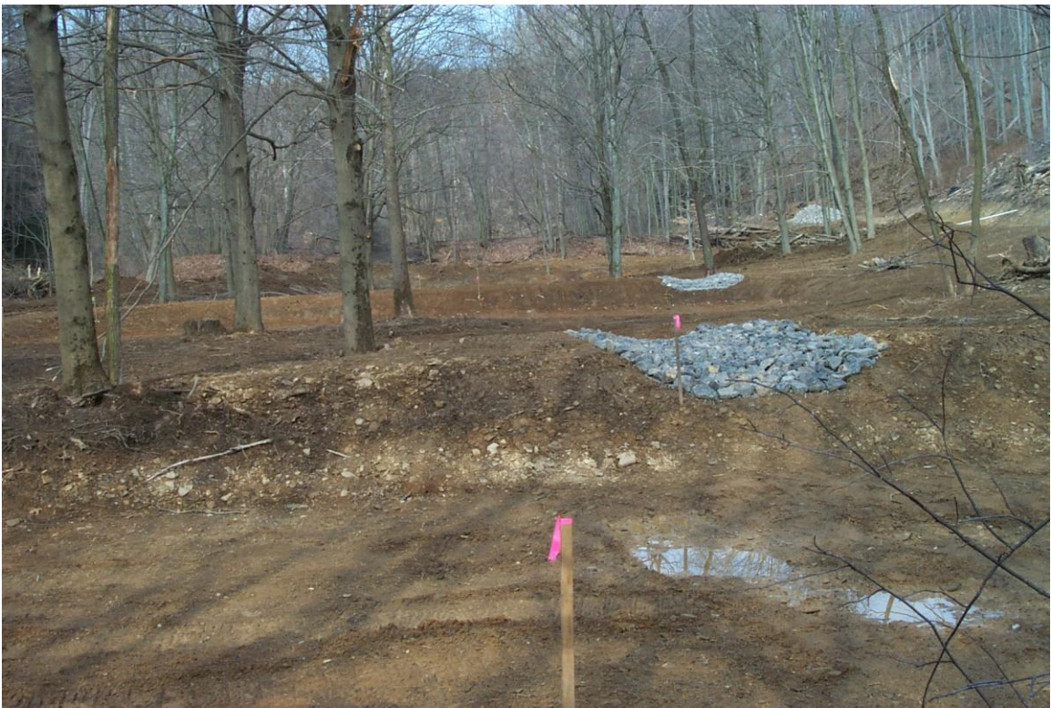
Picture 4: Construction of treatment cells showing transition channels
