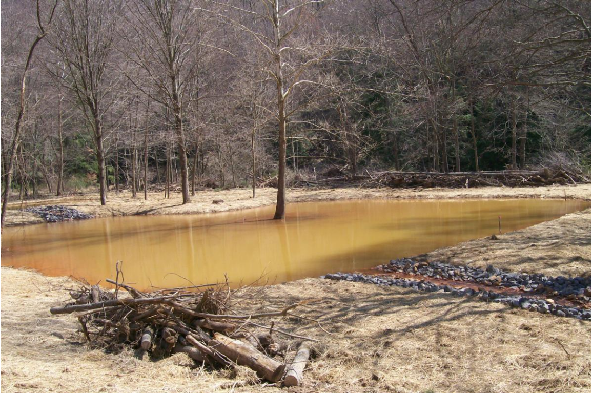
Picture 11: Finished second cell
