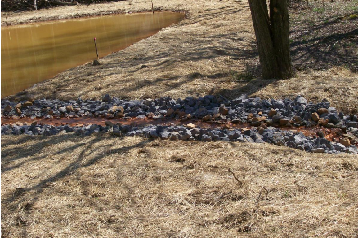
Picture 13: Detail of transition channel from second to third cell
