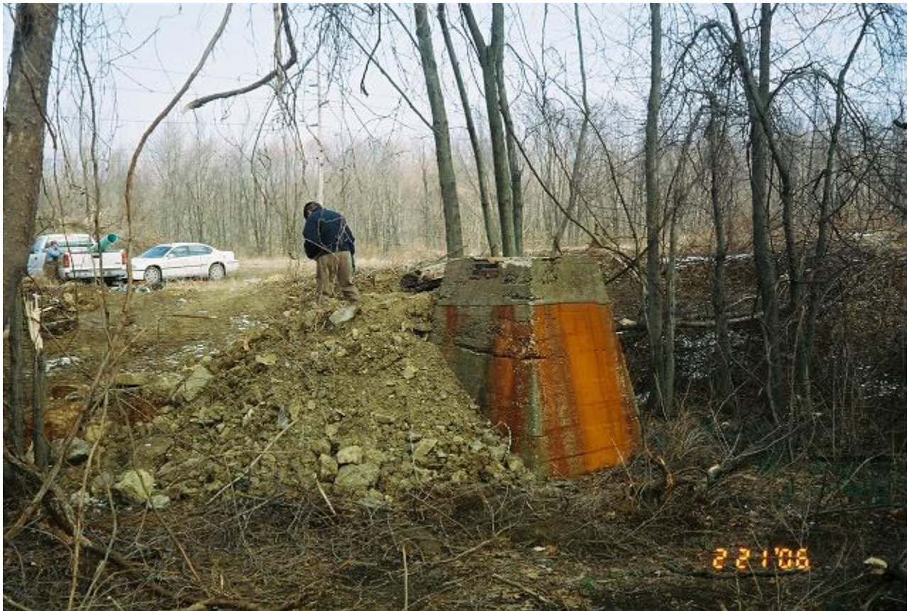
“Manhole” structure prior to sealing – note access ramp at left side
