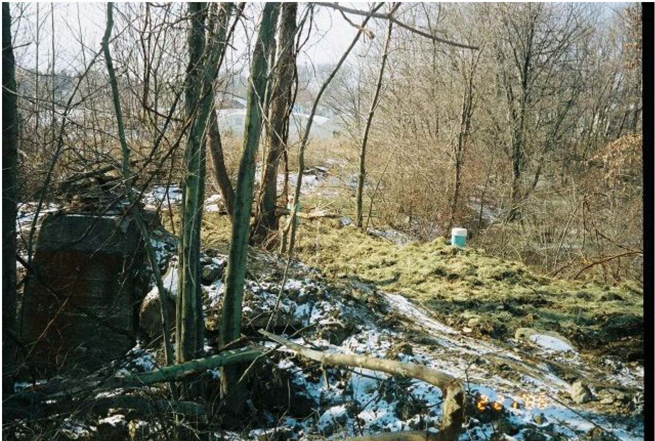
View from “Manhole” on left to Main Discharging Borehole Pipe, after fill and mulch placement
