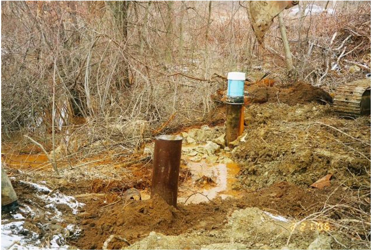
View of Main Discharging Borehole Pipe (with Fernco, stub and cap) and “Bubbler” with casing
