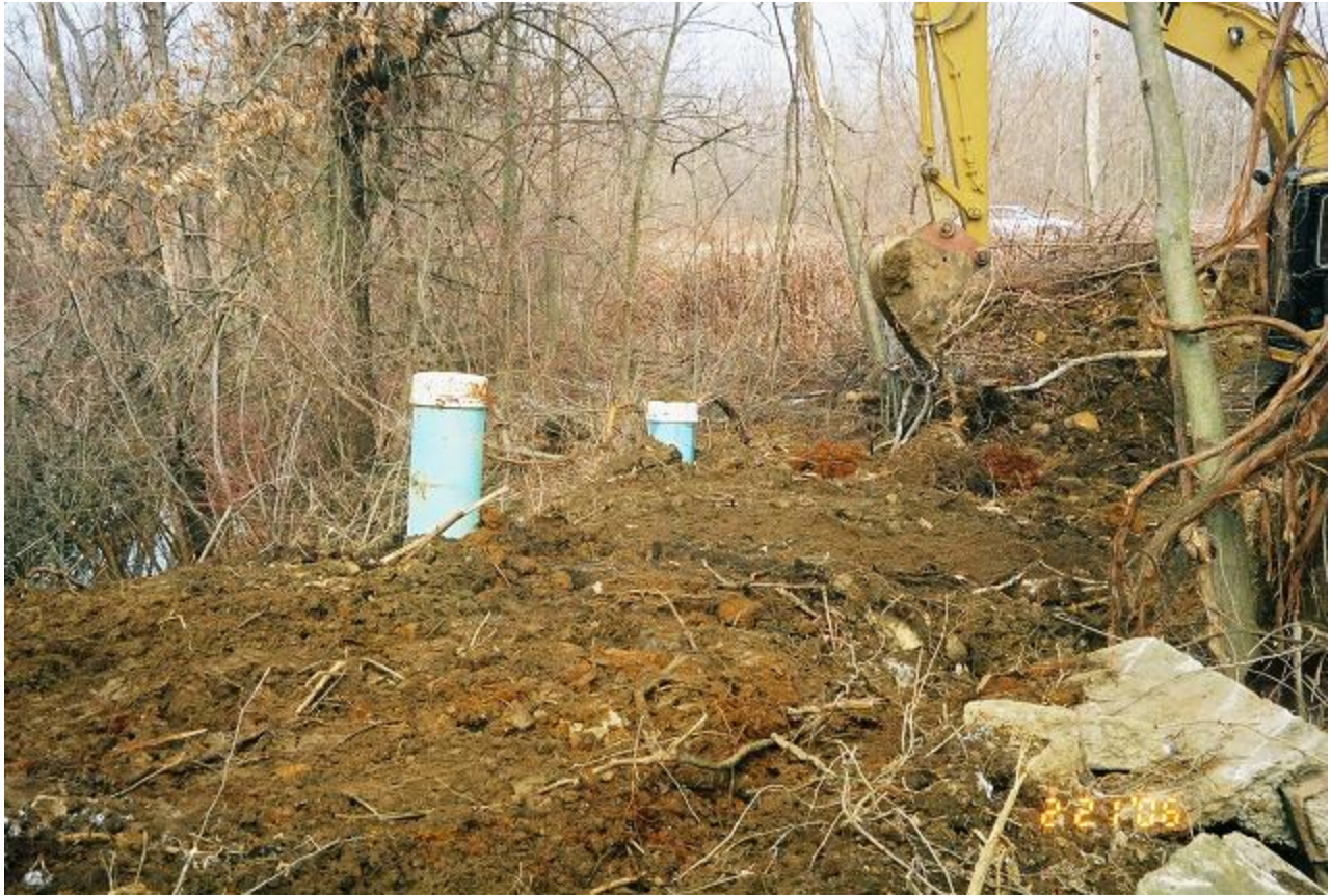
Main Discharging Borehole Pipe and “Bubbler” Pipe with caps and backfill
