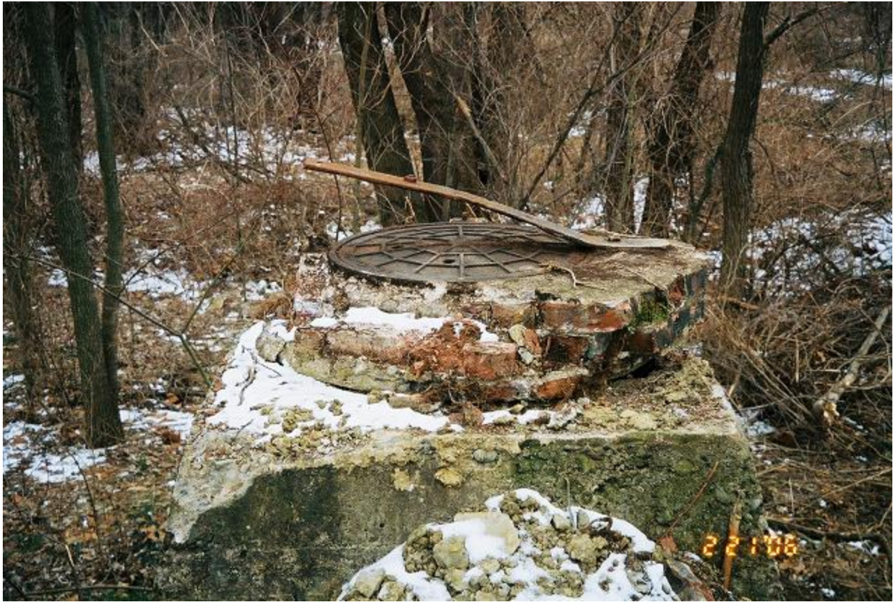
View of the “Manhole” structure with the lid set back in place
