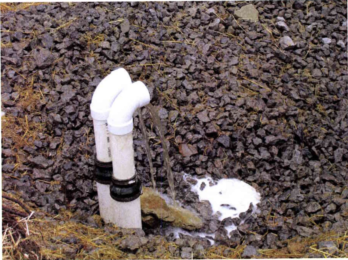
Discharge Piping and VFP Water Level Control
