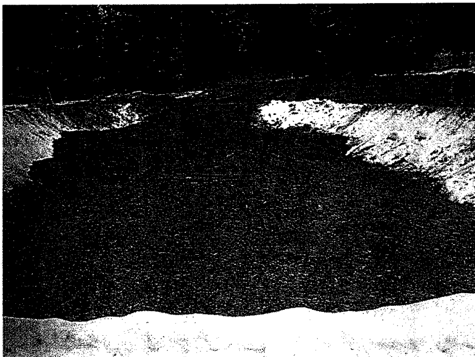
Mulch Covering Limestone in Both VFPs
