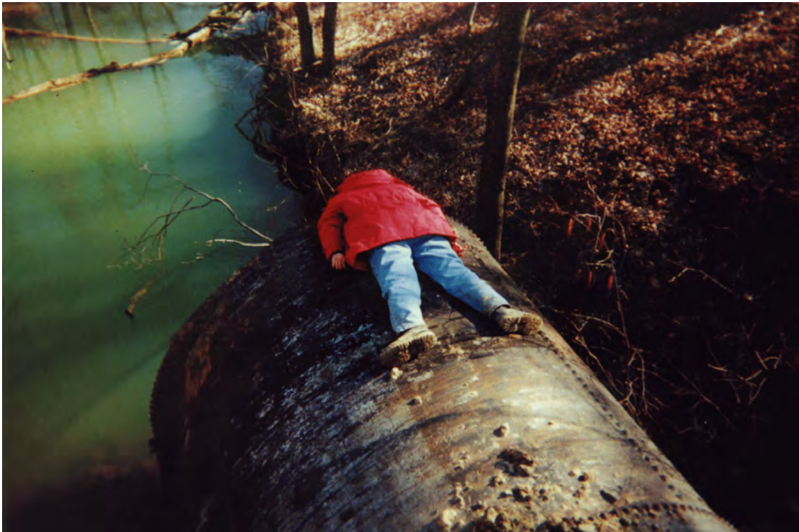
Margaret Dunn atop pipe after it had been placed for stream crossing.
