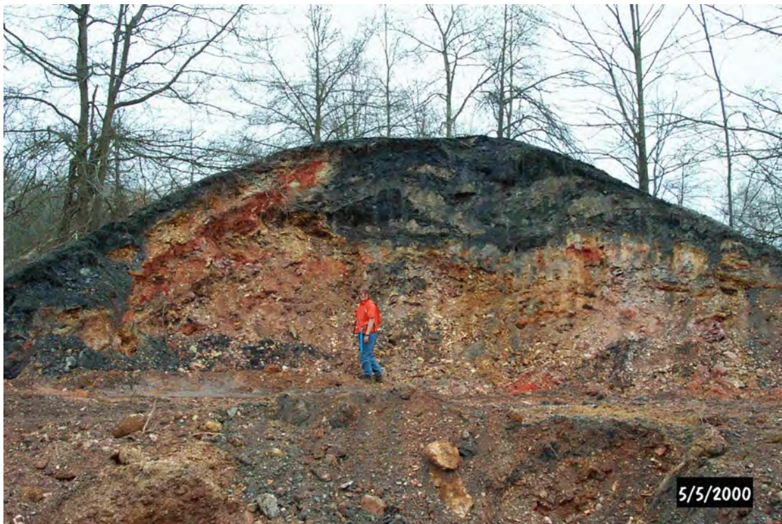
Cross-sections of refuse pile as seen during removal
