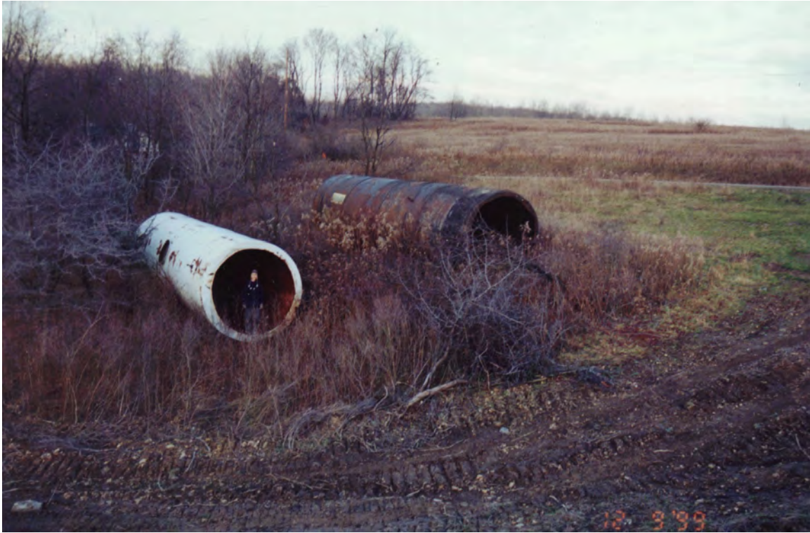
Two forty foot sections of pipe, seven feet in diameter, used for stream crossing. (Pictured: D. Peart)
