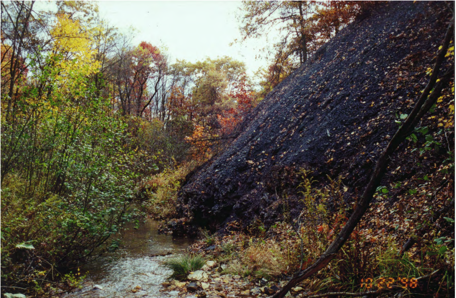
View of coal refuse pile looking downstream (south). Note toe of refuse extending into Murrin Run
