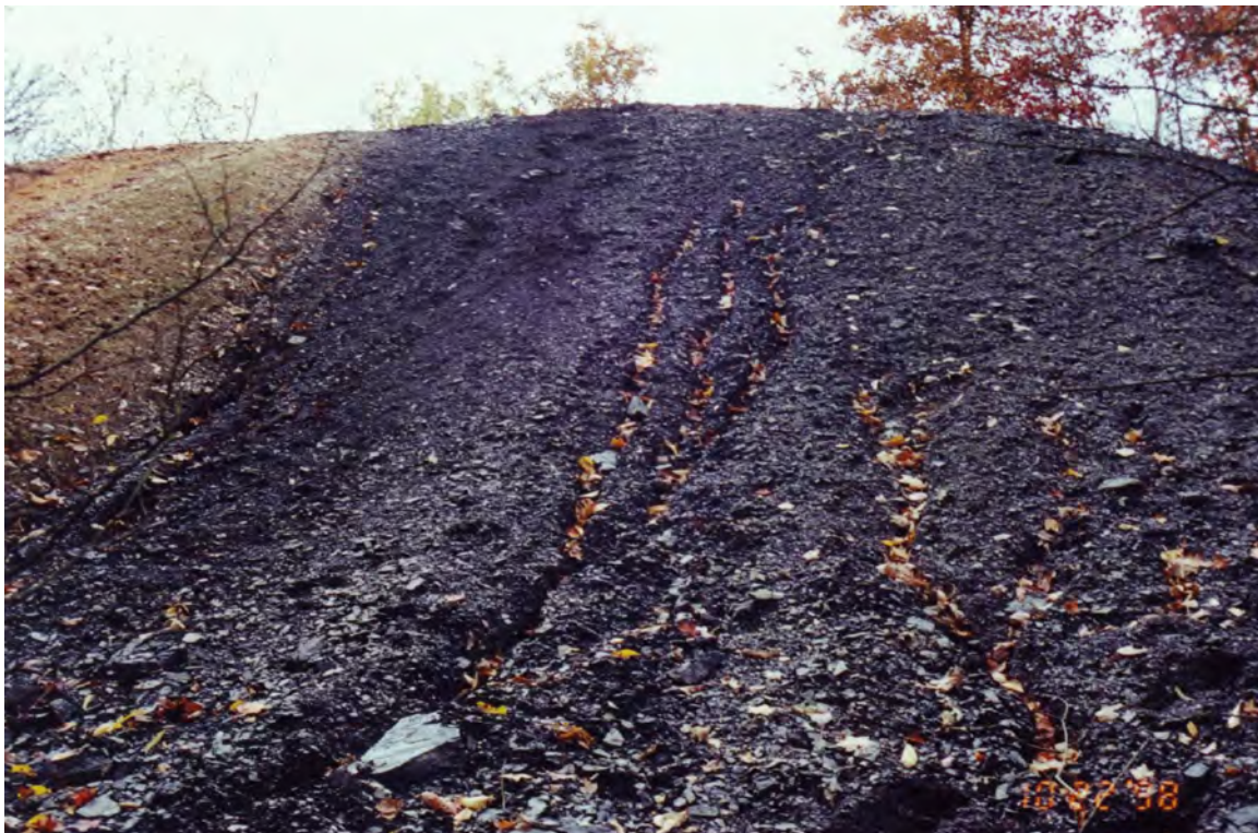
A portion of the 63,600 cy of coal refuse at the Goff Station Restoration Area. Fallen Leaves identify erosion gullies.
