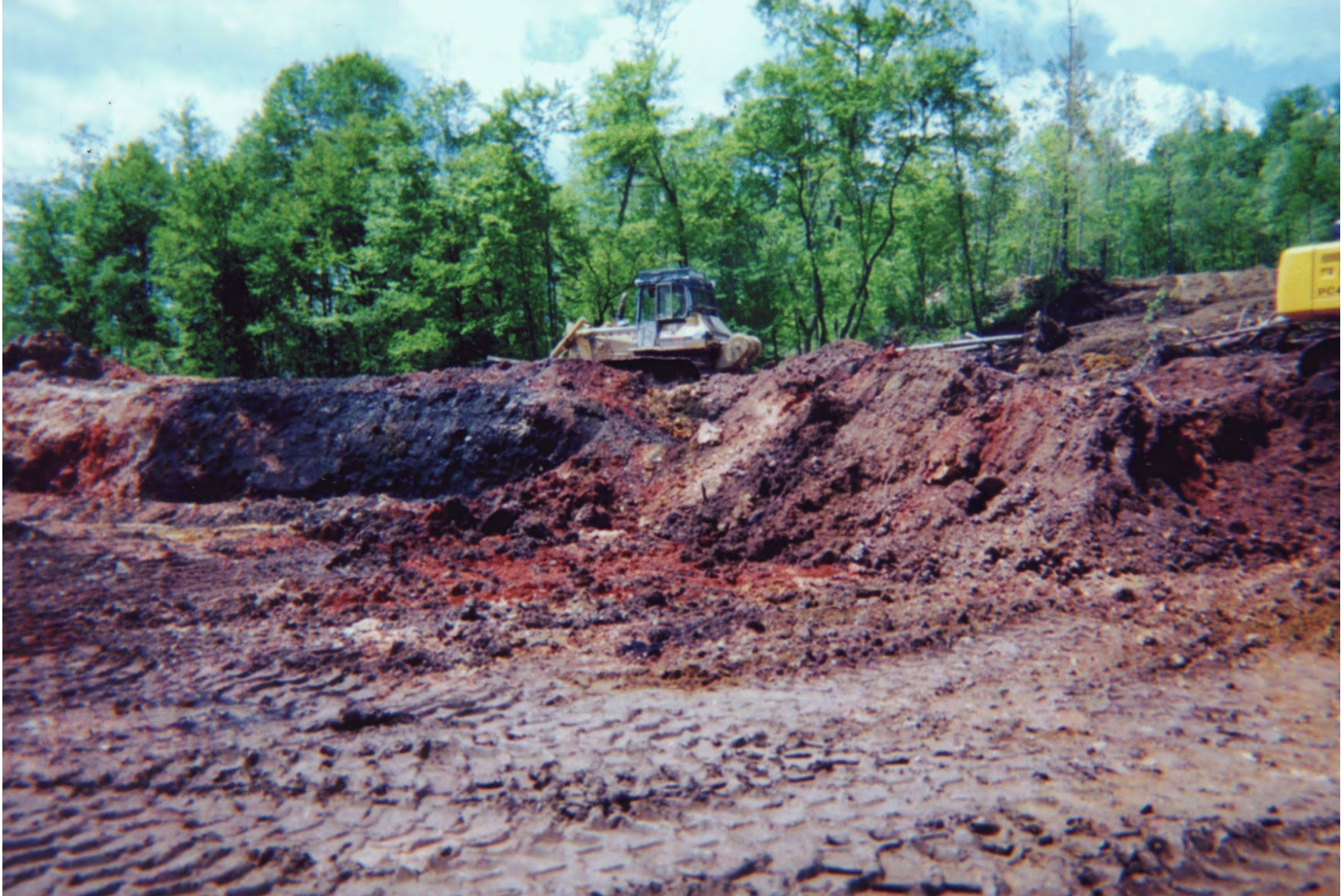
Bulldozer removing refuse at the Goff Station Restoration Area
