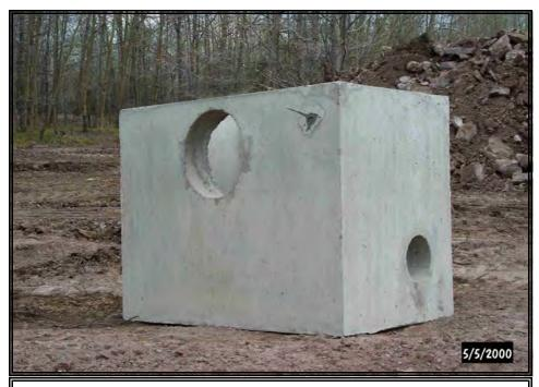
Inlet Control Structure: opening for piping from collection system (center) and one of two openings for piping to the Vertical Flow Ponds (right).
