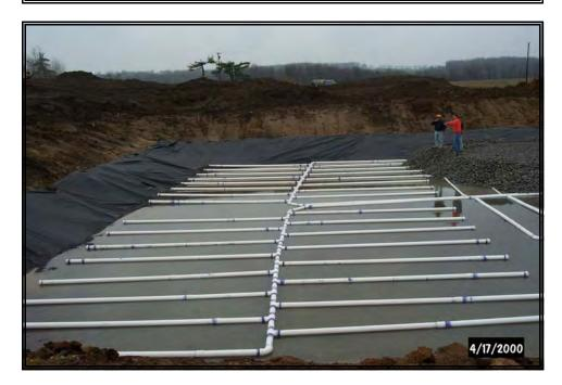
Vertical Flow Pond-North: lower underdrain tier of 4", perforated Sch. 40 PVC pipes on 4  $\frac{1}{2}$  -foot centers. Laterals plumbed into 4, 4", solid, Sch. 40 PVC mains, dividing pond into quadrants. Bedding stone  $\frac{1}{2}$  -foot of AASHTO #57 limestone.
