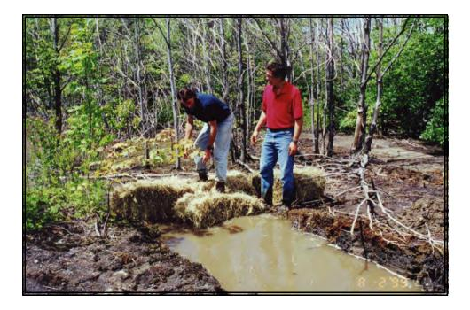
Installation of straw bales during temporary diversion of collected mine drainage from construction area. (8/2/99)
