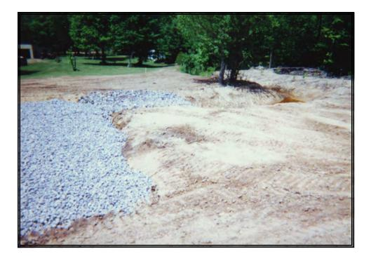
Horizontal Flow Limestone Bed: spillway to upgraded, preexisting channel to Seaton Creek tributary. Outlet pipe from manifold not visible. (5/26/00)
