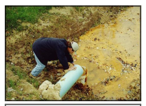
Tim Gillen, PG, Knox DMO, measuring discharge flow prior to passive system installation. (10/22/99)
