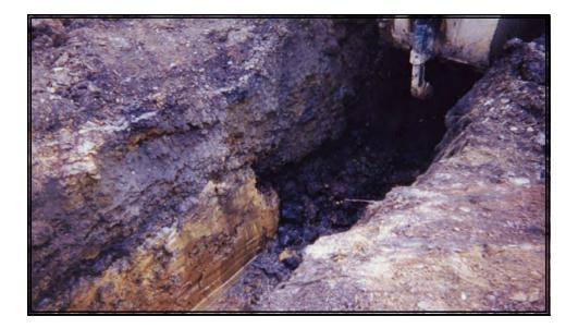
Interceptor trench for abandoned mine drainage. Water ponded behind clay barrier in coaly spoil material. (8/2/99)
