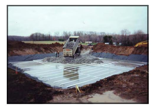
Vertical Flow Pond-North: AASHTO #1 limestone placed above lower underdrain tier. Note grade stakes and geotextile extending onto embankments. (4/17/00)
