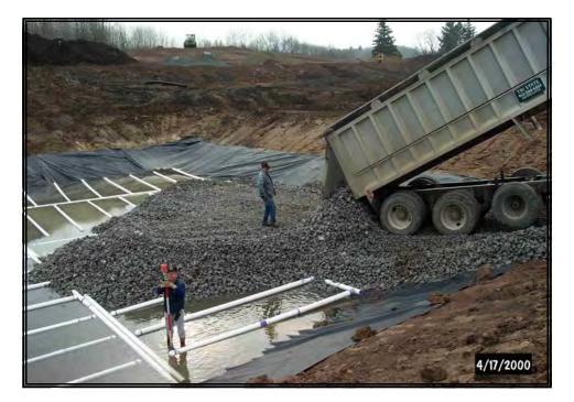
Vertical Flow Pond-North: AASHTO #1 limestone placed above lower underdrain tier. Note rodman surveying for "As-Builts."
