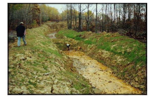
Pipe installed in temporary interceptor trench to monitor discharge. (10/22/99)
