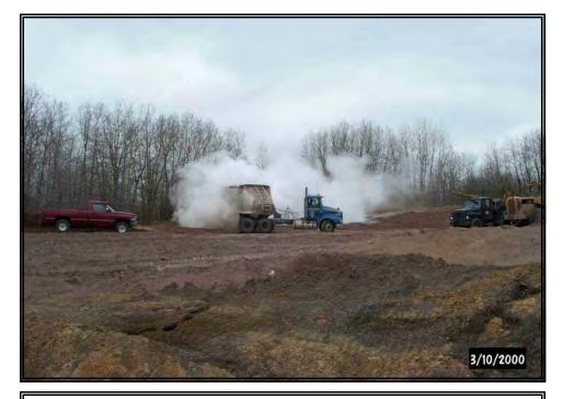
Steam rising during delivery of alkaline, circulating, fluidized-bed coal ash from the Scrubgrass Generation Plant, Kennerdell, PA. 35,000 tons were used to reclaim a barren portion of the upland spoil area.
