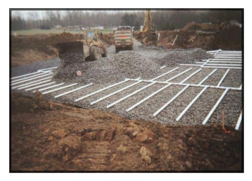
Vertical Flow Pond-North: AASHTO #1 limestone placed above upper underdrain tier. Note coordinated effort with tri-axle delivering stone, rubber-tired, front-end loader spreading stone, and excavator constructing trenches for outlet pipes. (4/17/00)
