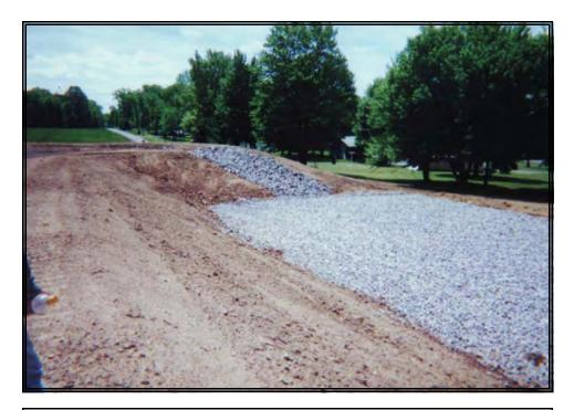
Horizontal Flow Limestone Bed: spillway from wetland stabilized with R4 limestone rip rap. (5/26/00)
