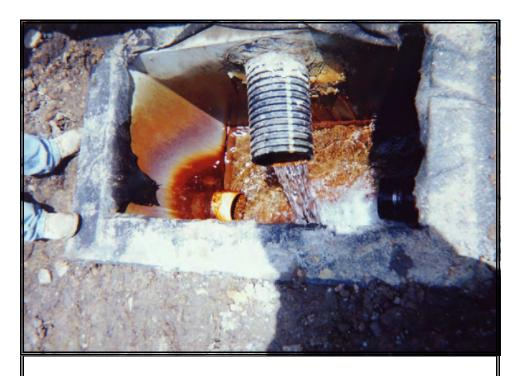
Inlet Control Structure after installation. 8", solid, N12 piping conveying flow from Anoxic Collection System. Two, 6", solid, Sch. 40 PVC pipes: pipe to Vertical Flow Pond-North (left) and - South (right). (5/26/00)
