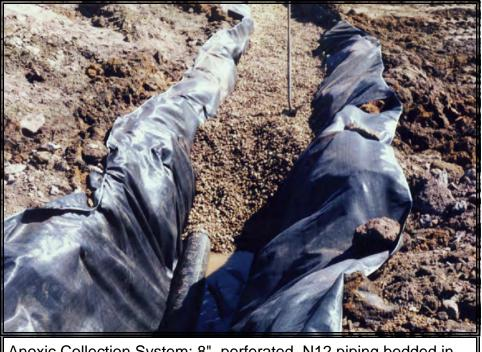
Anoxic Collection System: 8", perferated, N12 piping bedded in gravel and wrapped in woven drainage geotextile. (4/5/00)
