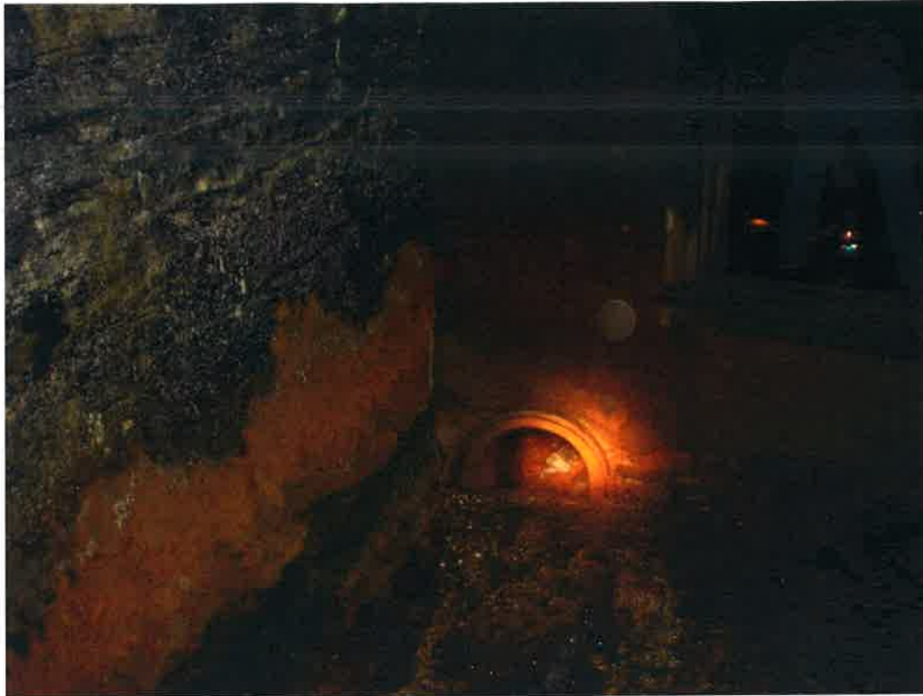
Figure 11. The “Lucerne 3A Mine Discharge” exiting the Campbell Mine and piped underneath the man mover to surface.
