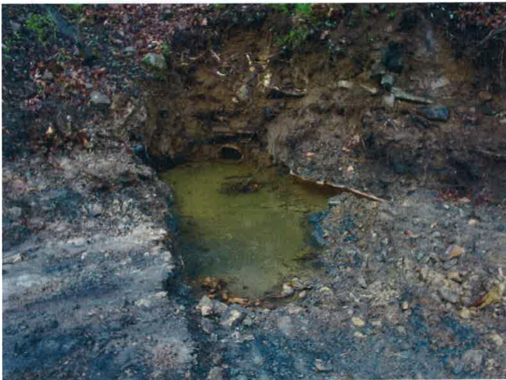
Figure 9. The pipe exiting the Lucerne 3A Mine Portal, the true origination point.
