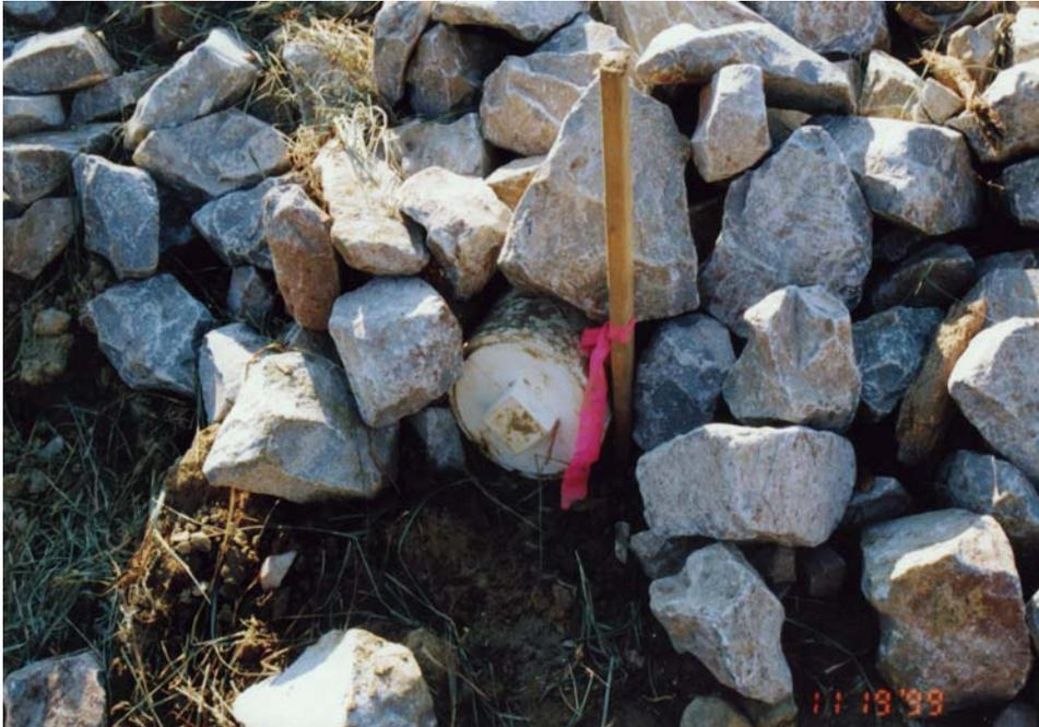
6" Bottom flush pipe for Vertical Flow Pond. (11/19/99)
