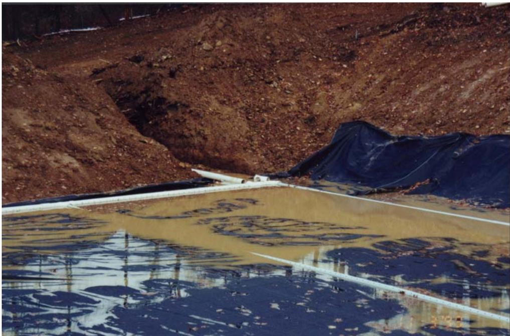
Effluent pipe of Vertical Flow Pond leading to Settling Pond #2. (11/2/99)
