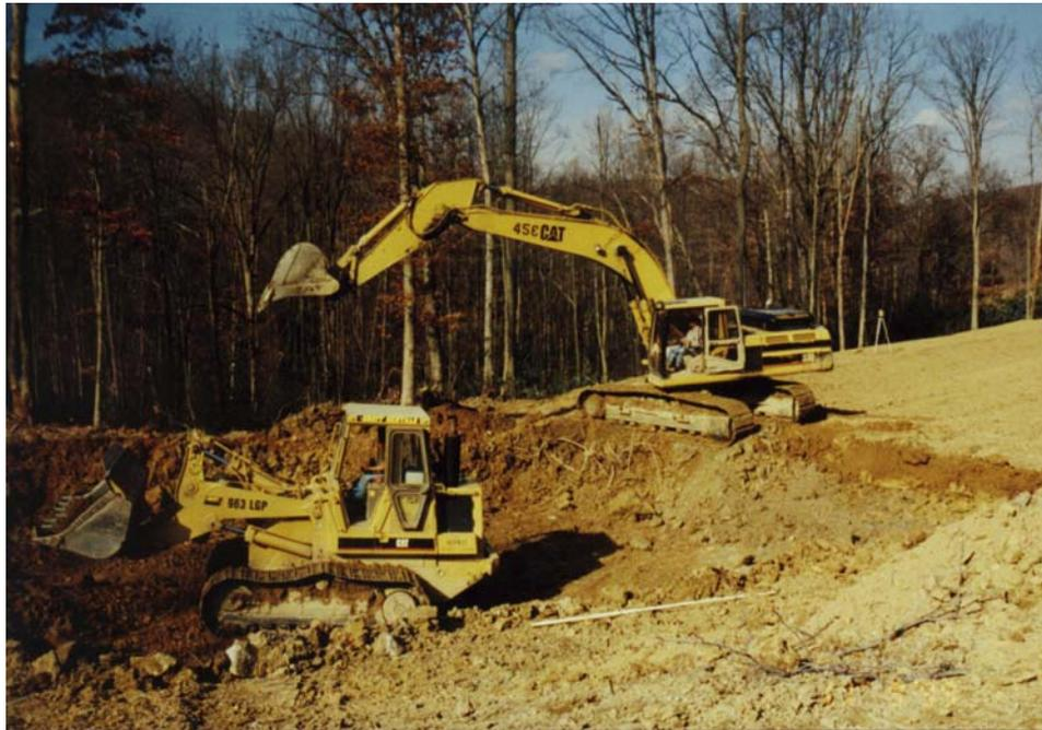
Construction of 500 ton Horizontal Flow Limestone Bed.
