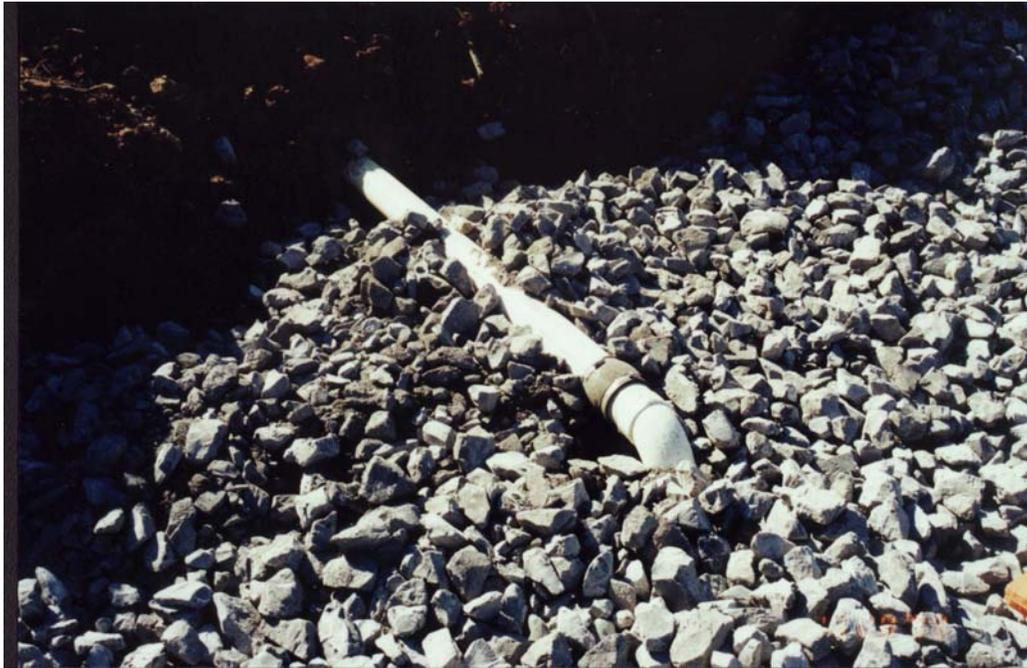
Influent pipe from Anoxic Collection System to Anoxic Limestone Drain. (10/28/99)
