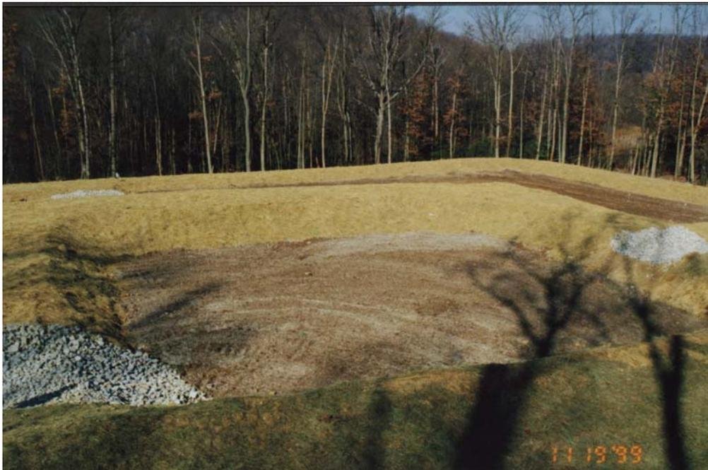
Completed Vertical Flow Pond with 600 tons of AASHTO#1 overlain by mixture containing 36 tons of spent mushroom compost, 71 tons of AASHTO #57, 69 tons of AASHTO #10 aggregate. (11/19/99)
