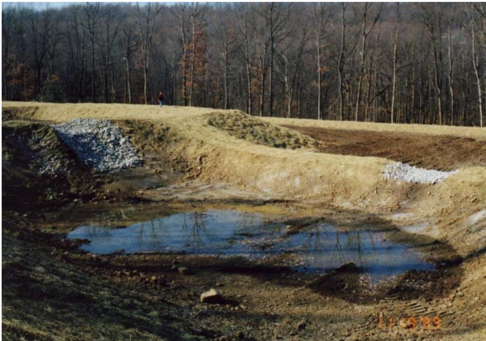
Settling Pond #2 before water began flowing through the passive treatment system. (11/19/99)
