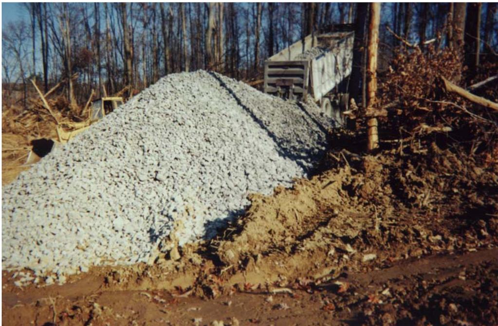
AASHTO #1 limestone used in the construction of the ALD and VFP. (10/29/99)
