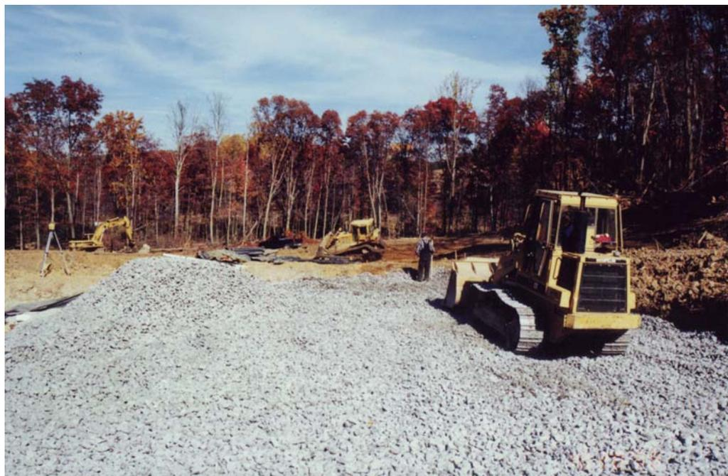
Construction of Anoxic Limestone Drain (670 tons), part of the Phase I passive treatment system. (10/28/99)
