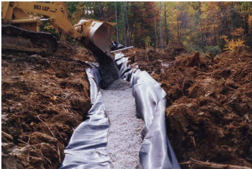
Placing of sandstone aggregate in collection ditch. (10/11/99)
