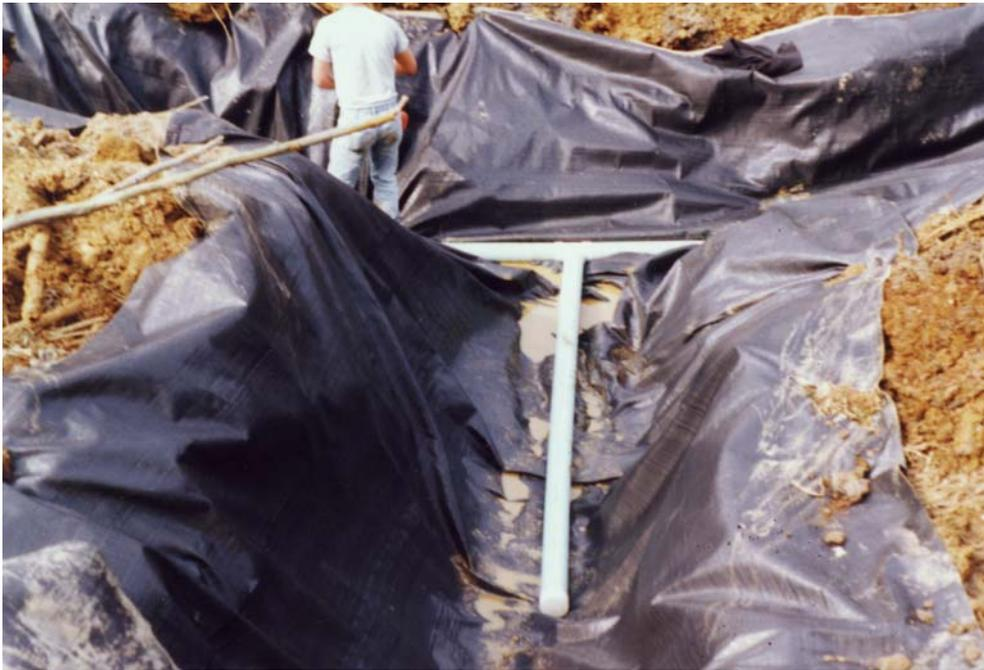
4 inch, perforated SDR 35 pipe in collection system. One of two laterals shown. (10/11/99)
