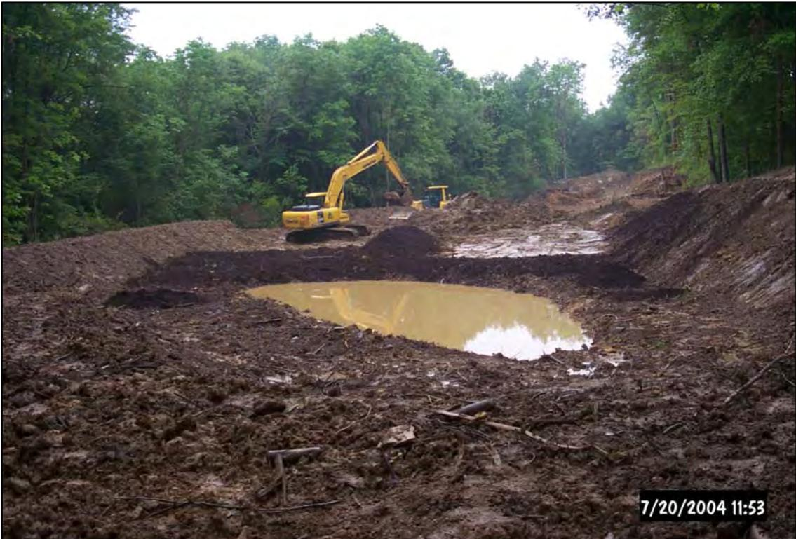
Excavator constructing berm in the area of the BC19 discharge to direct flows to the drop structure visible in the foreground.
