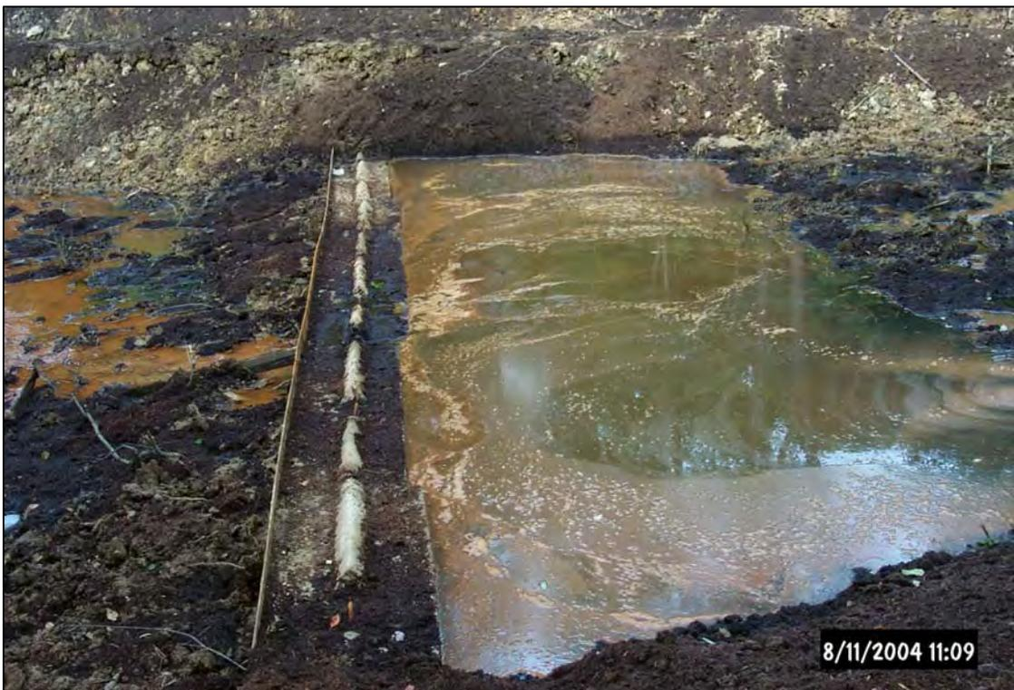
Drop structure and level spreader. The level spreader maintains consistent water levels within the main basin of the treatment wetland and creates an aerating sheet flow to the lower portion of the treatment wetland. This and other drop structures slow water velocities and allow for accumulation of metal precipitates.
