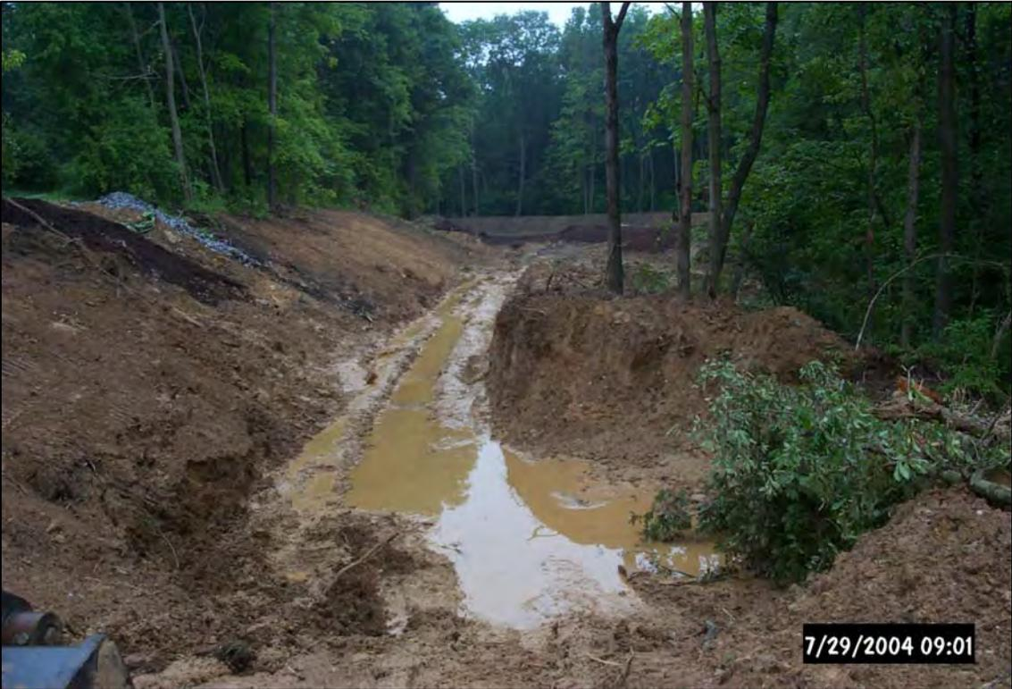
Plunge pool near the BC19B discharge and the bioswale conveying flows to the main basin of the treatment wetland.
