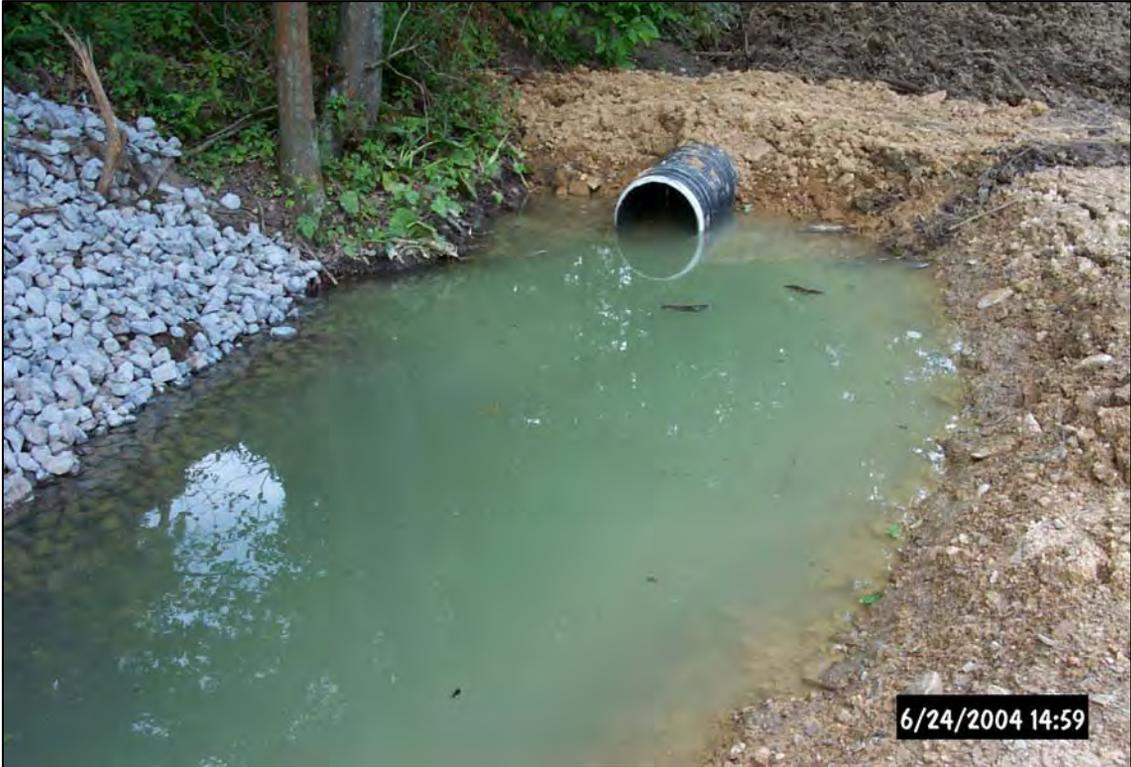
Plunge pool and culvert for diversion of surface flows from passive treatment system.
