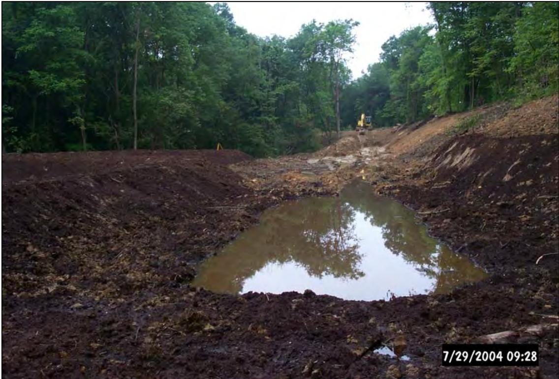
Plunge pool in the main basin of the treatment wetland near the end of the bioswale that conveys flows from the BC19B discharge.
