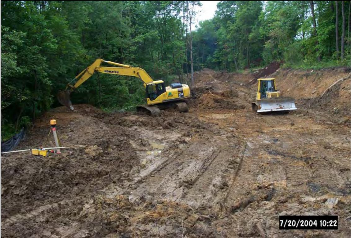
Wetland basin and berm construction near outlet and end of bioswale. Laser level and stadia rod utilized to maintain grades throughout construction.
