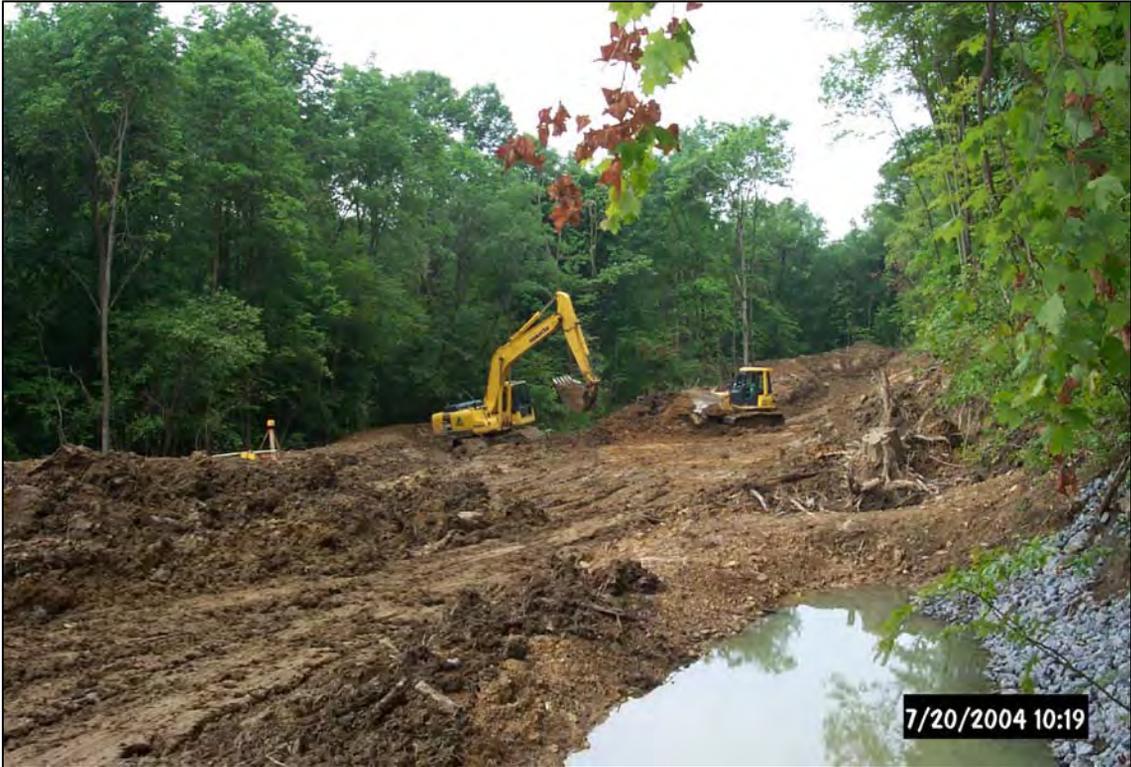
Plunge pool for surface water diversion in foreground. In background, earth moving with bulldozer and excavator in the area near the wetland outlet and berm of the bioswale.
