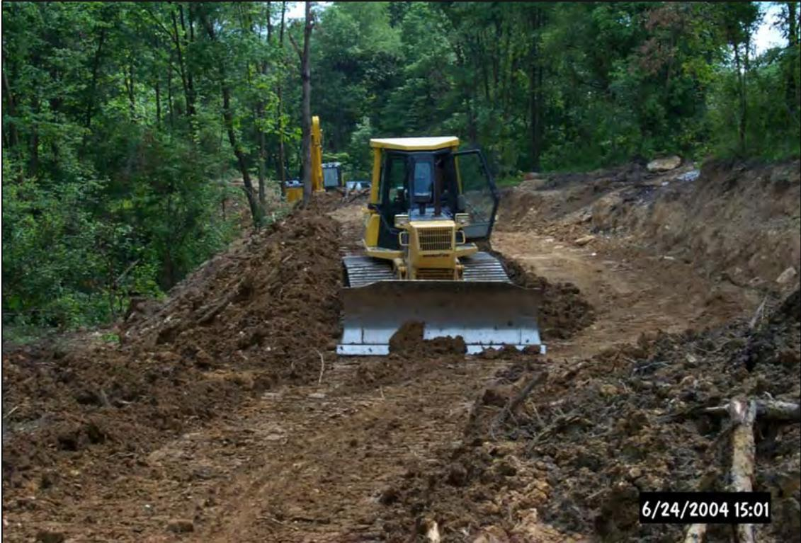
Early earth moving with bulldozer in area of the bioswale and berm.
