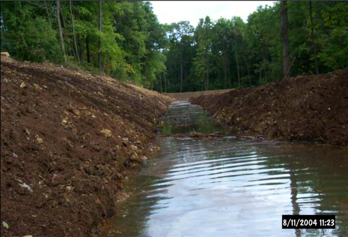
Bioswale conveying flows from the BC19B discharge to the main basin of the treatment wetland.
