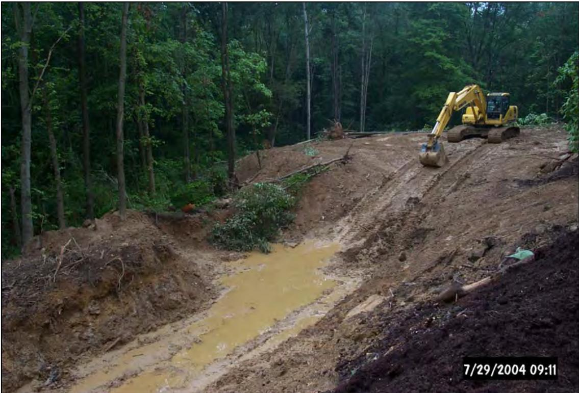
Excavator grading slope south near the drop structure for the BC19B discharge.
