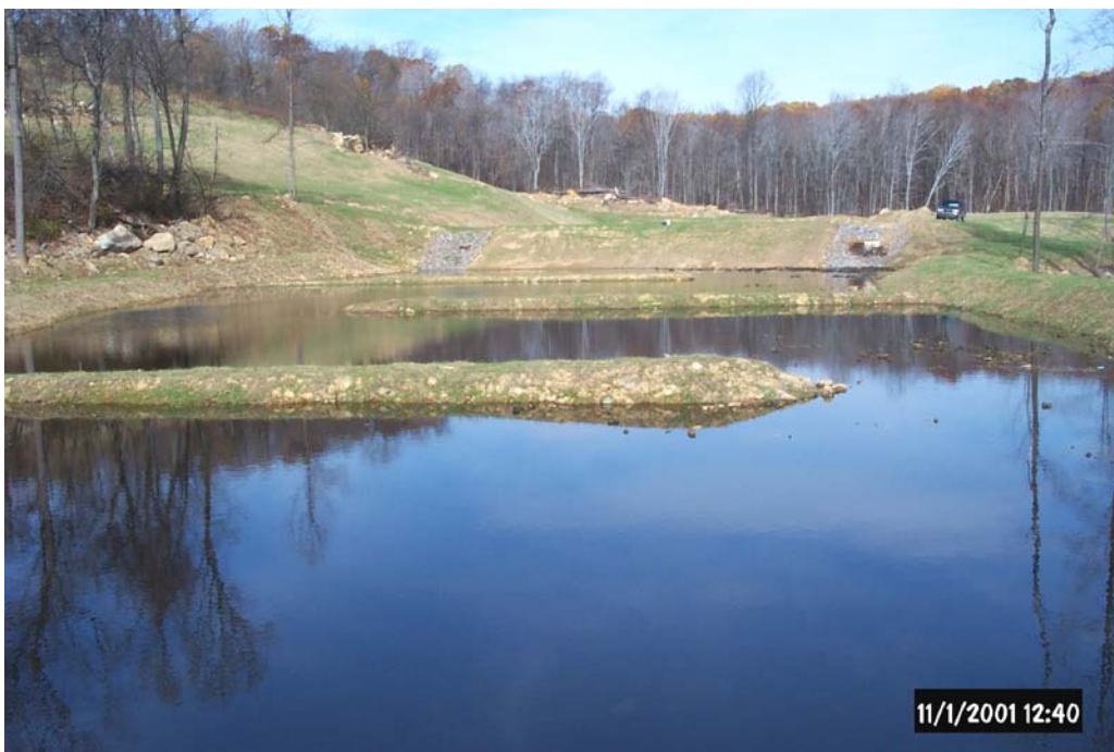
Views of the unplanted wetland, which the effluent of the Vertical Flow Ponds enters for further oxidation and precipitation of metals.
