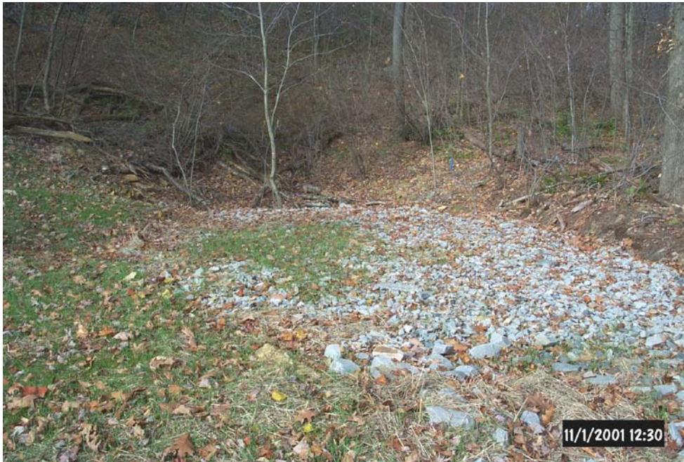
Former location of mine drain, which is now utilized as part of the collection system and covered with limestone.
