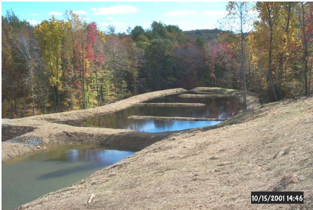
Views of the unplanted wetland, which the effluent of the Vertical Flow Ponds enters for further oxidation and precipitation of metals.
