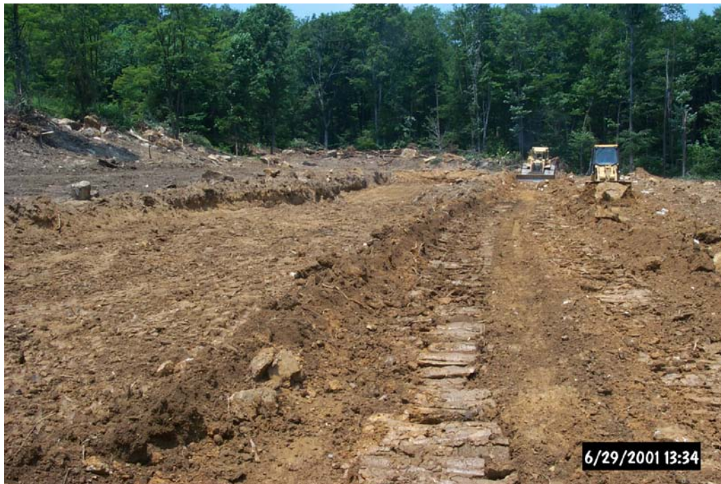
Construction of the Vertical Flow Ponds at the Laurel Run North Passive Treatment System by Amerikohl Mining Inc.
