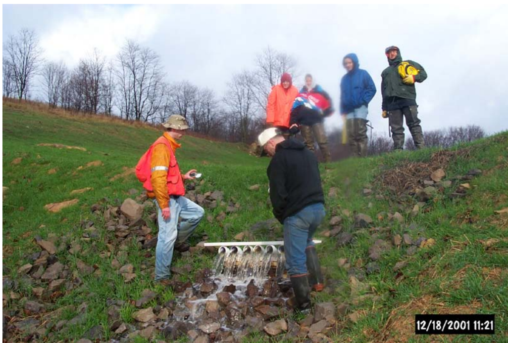
Shaun Busler, BioMost, Inc (left) with volunteer Terry Frombach (right) "burp" the system and balance flows from a Vertical Flow Pond while PA DEP interns look on from behind.
