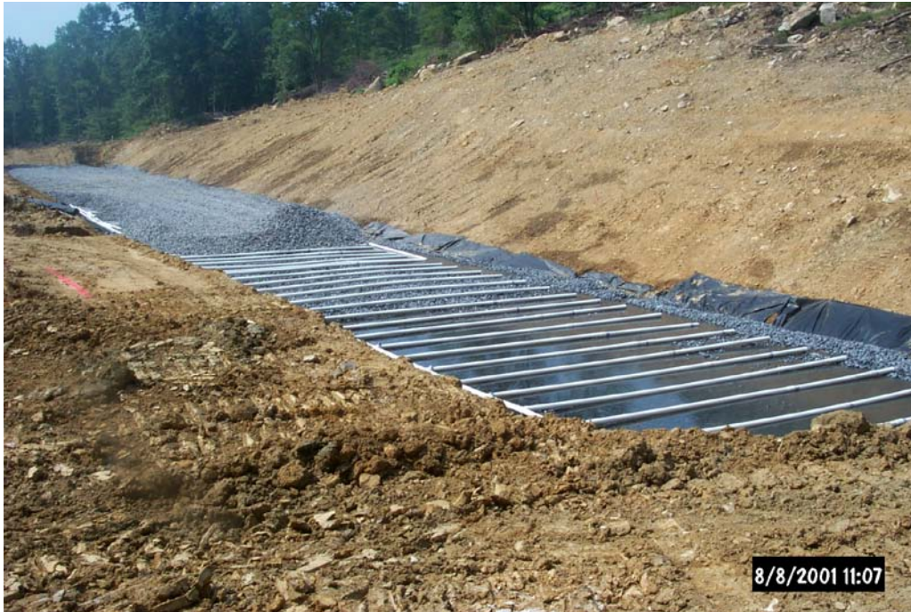
Vertical Flow Pond under construction. Note the underdrain piping system and a portion of the second layer of limestone put in place.
