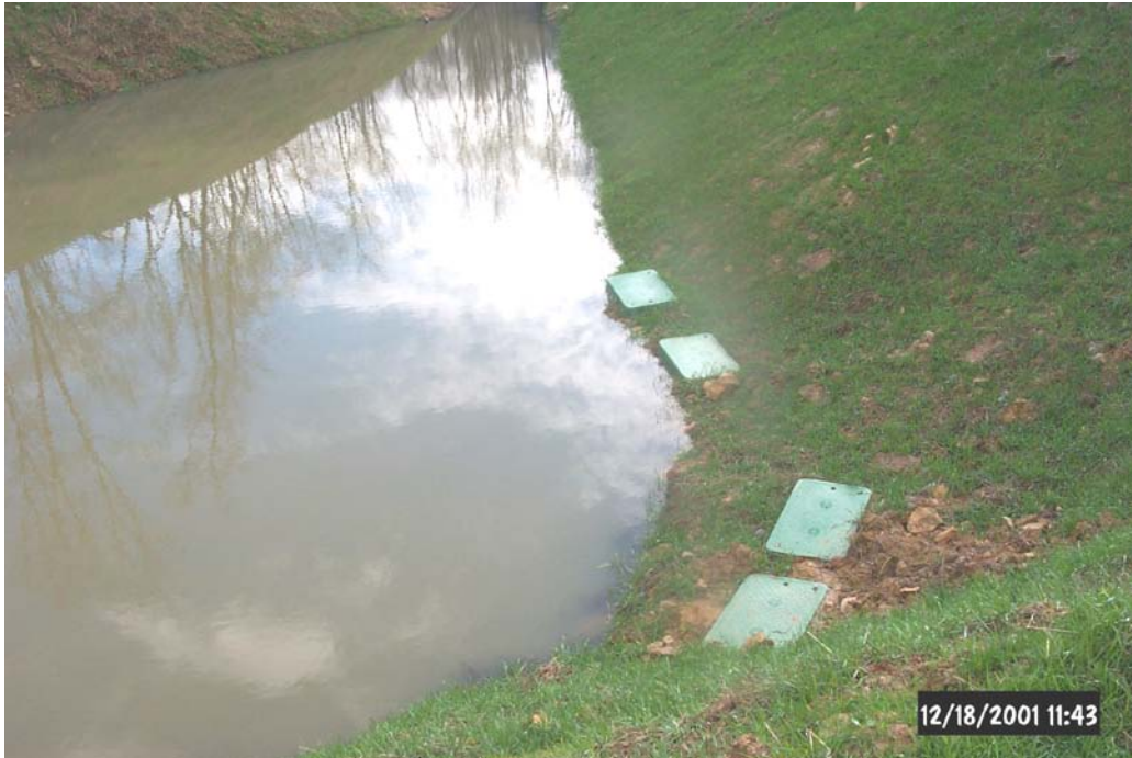
Flush pond and valve boxes for the flush pipes of the Vertical Flow Ponds.
