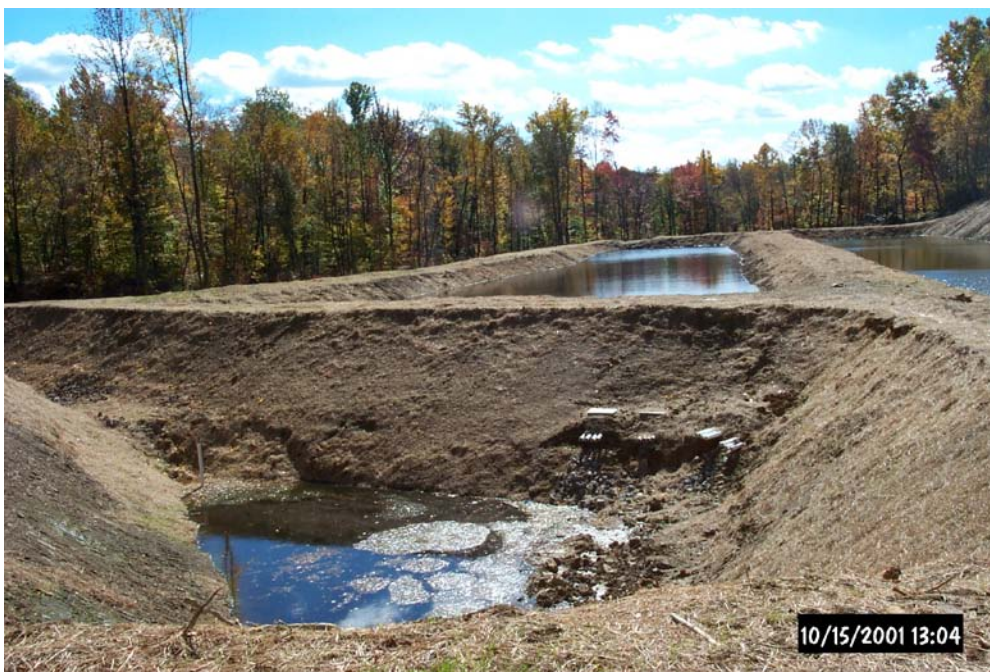
Flush Pond in the foreground is used as a holding pond during flushing events of the Vertical Flow Ponds behind it.
