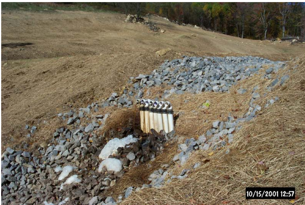
Peripipe discharge pipes for the Vertical Flow Ponds allow for easy balancing, control, and adjustments to flow rates within the ponds.
