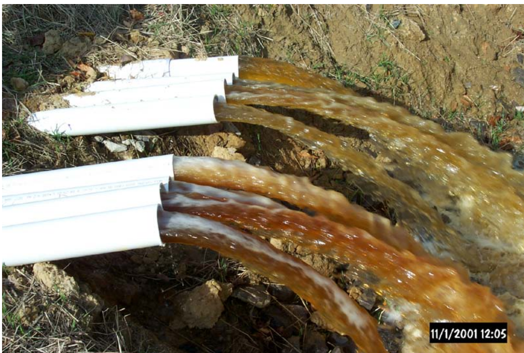
A flushing event only a couple of months after the passive treatment system was placed on line.
