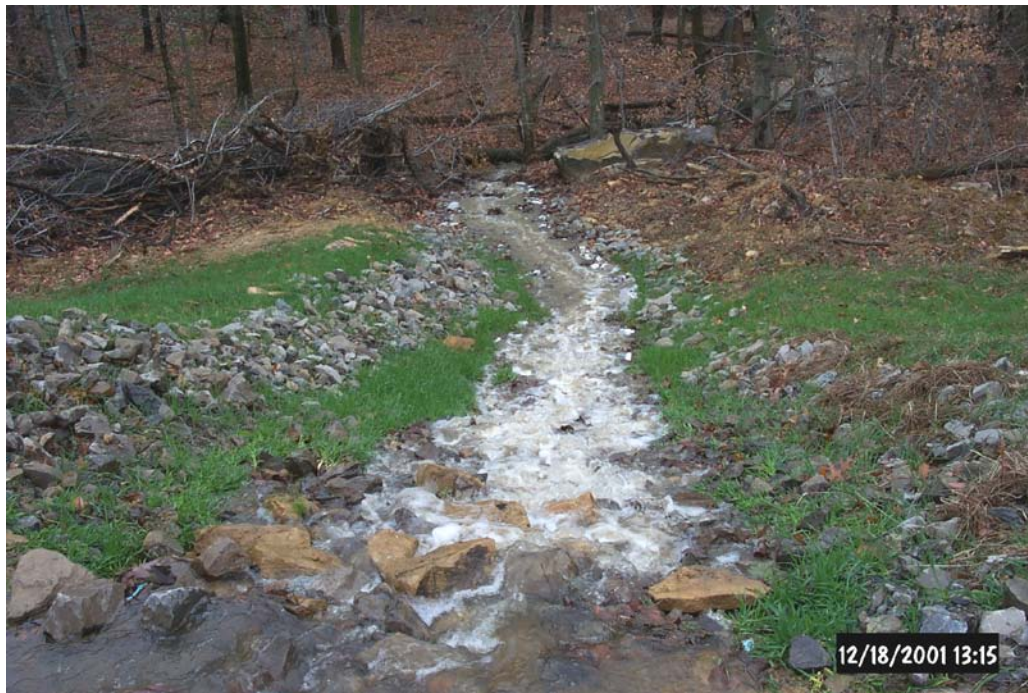
Final effluent from the passive treatment cascading down the rip-rap lined spillway to enter Laurel Run.
