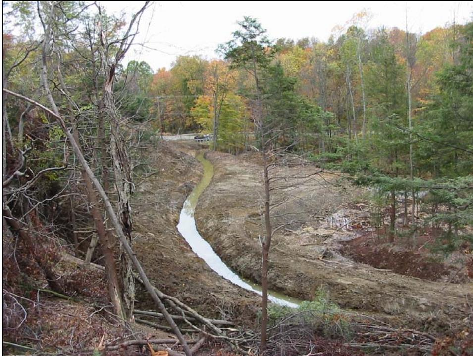
A post-construction view from the diversion ditch on the hilltop above Fox Run shows the newly installed channel that conveys the mine water (above). In the lower picture you see the end of the channel emptying into the settling pond and part of the wetland area. The site was timbered by the landowner with non-marketable treetops later placed in windrows for wildlife.
