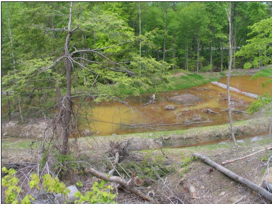
The settling pond water flows through a limestone aggregate spillway to aerate and distribute the mine drainage evenly prior to entering the wetland area.
