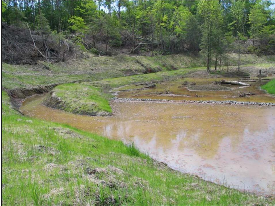
Suspended solids are retained in the settling pond where the water slows down before crossing the spillway.
