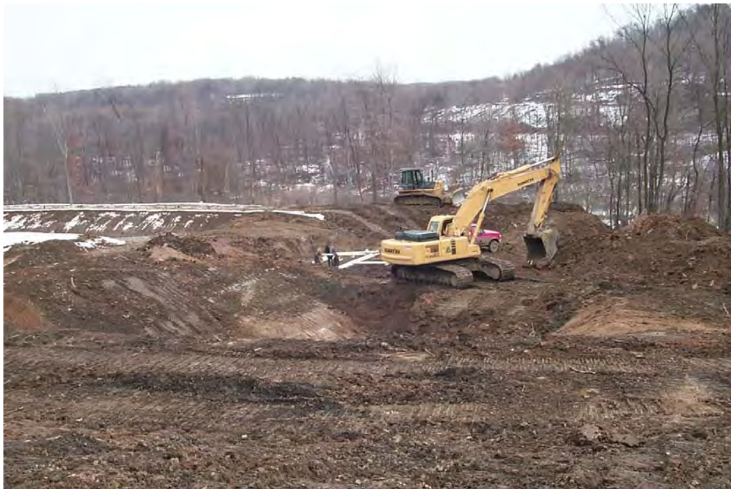
Quality Aggregates constructing Vertical Flow Ponds #3 & #4 of the ST 40/40A/42 system.
