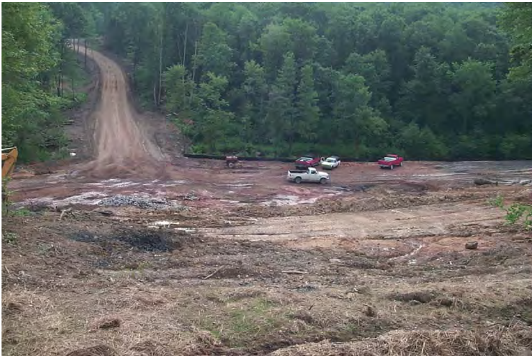
Gob removal largely completed. (6/26/00)
