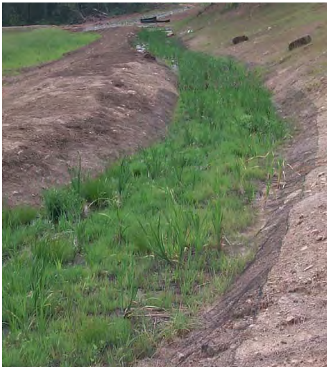
Growth in Bioswale after approximately 8 weeks. (8/16/01)
