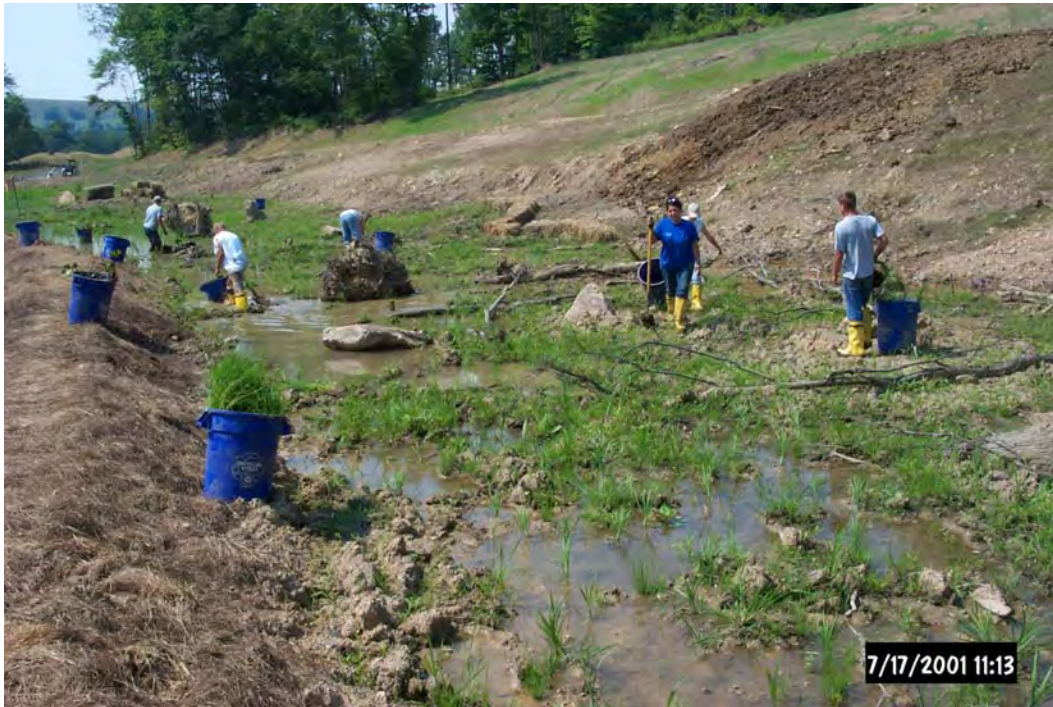
Final polishing wetland being planted by youth from the Butler County Juvenile Court Services WORC program.
