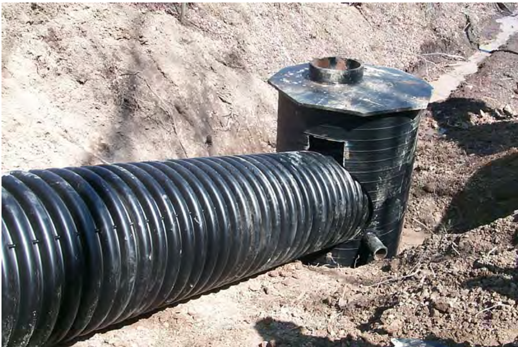
Installation of tunnel onto the bat hibernaculum. (4/4/01)
