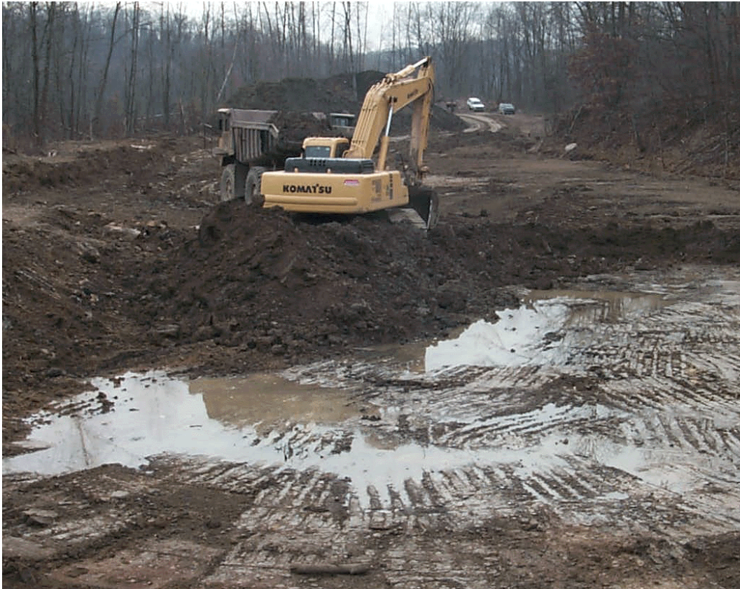
Placement of hydric substrate in ST41 Upper Wetland. (11/8/00)
