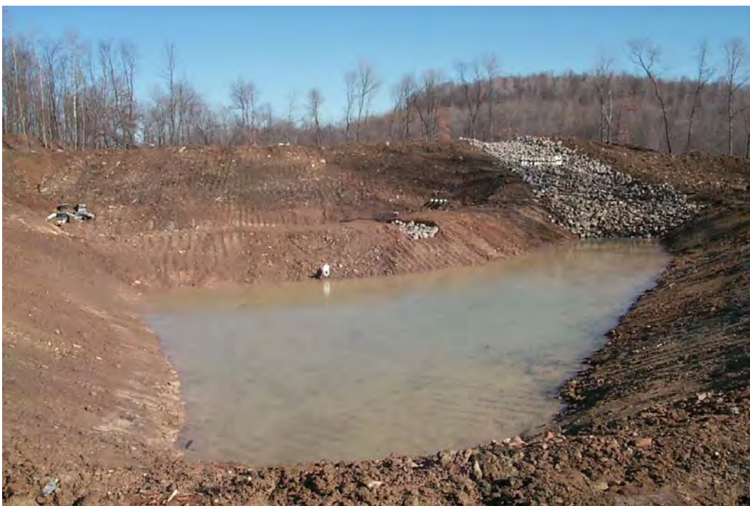
View of ST40/40A/42 System Wetland 2 after construction before planting.
