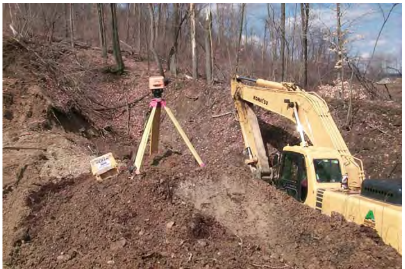
Stadia rod and laser level used to set the hibernaculum and tunnel to appropriate depth and slope. (3/23/01)
