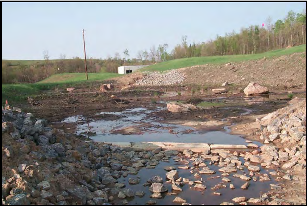
ST 38/39 wetland with following installation of new outlet structure. (5/7/01)
