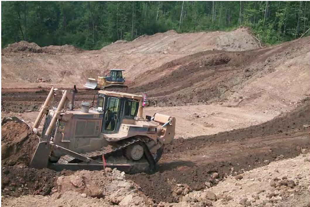
Quality Aggregates constructing ST38/39 Vertical Flow Ponds #1 & #2 which operate in parallel.
