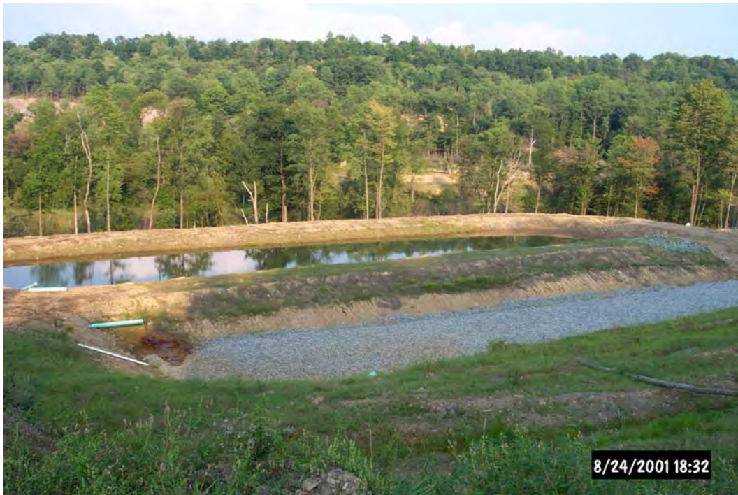
View of ST40/40A/42 Vertical Flow Ponds #3 & #4.
