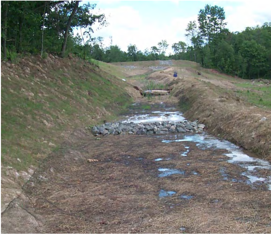
Installation of netting in Bioswale completed before transplanting wetland plants. (7/13/01)
