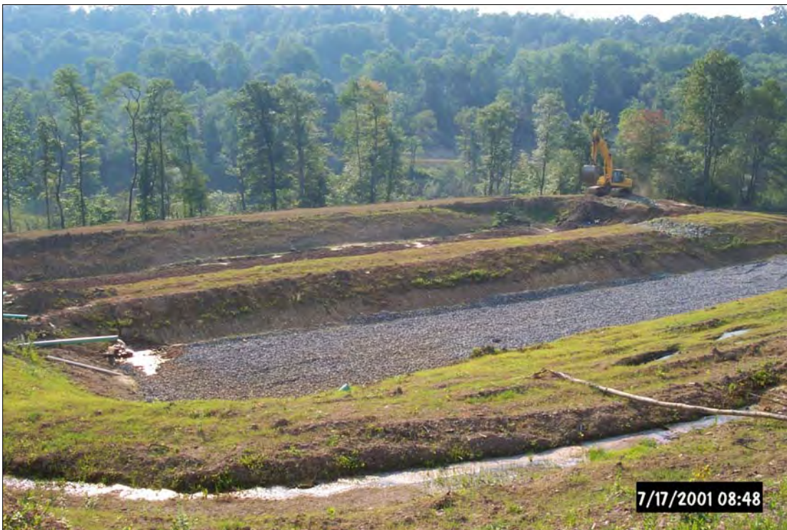
Vertical Flow Ponds # 3 and #4 under construction.
