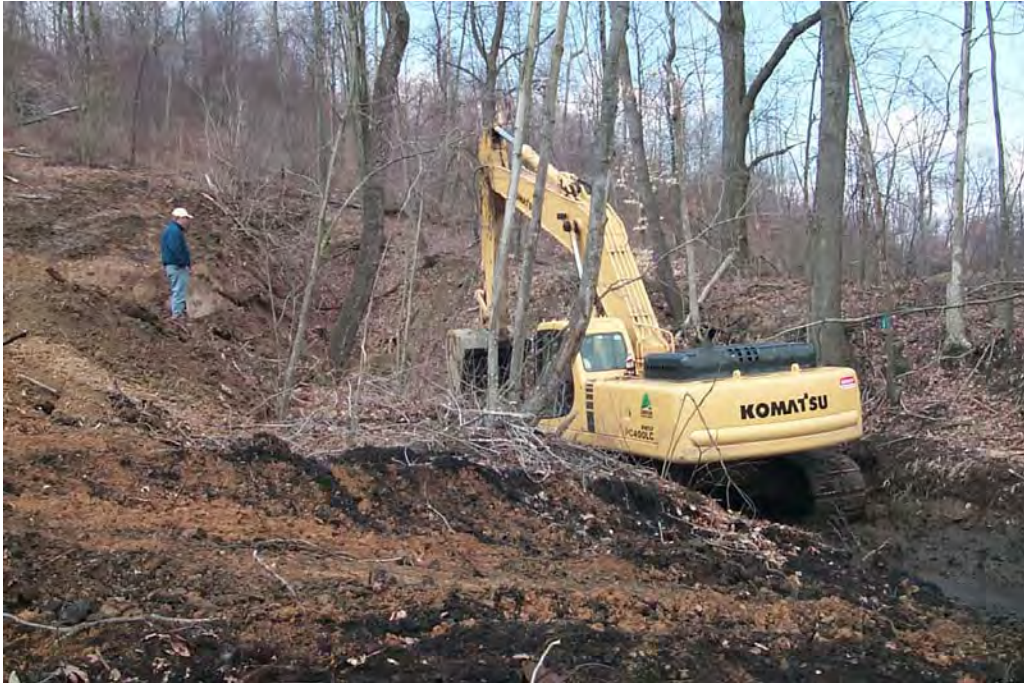
Excavation begins for placement of the hibernaculum within the ravine. (3/23/01)
