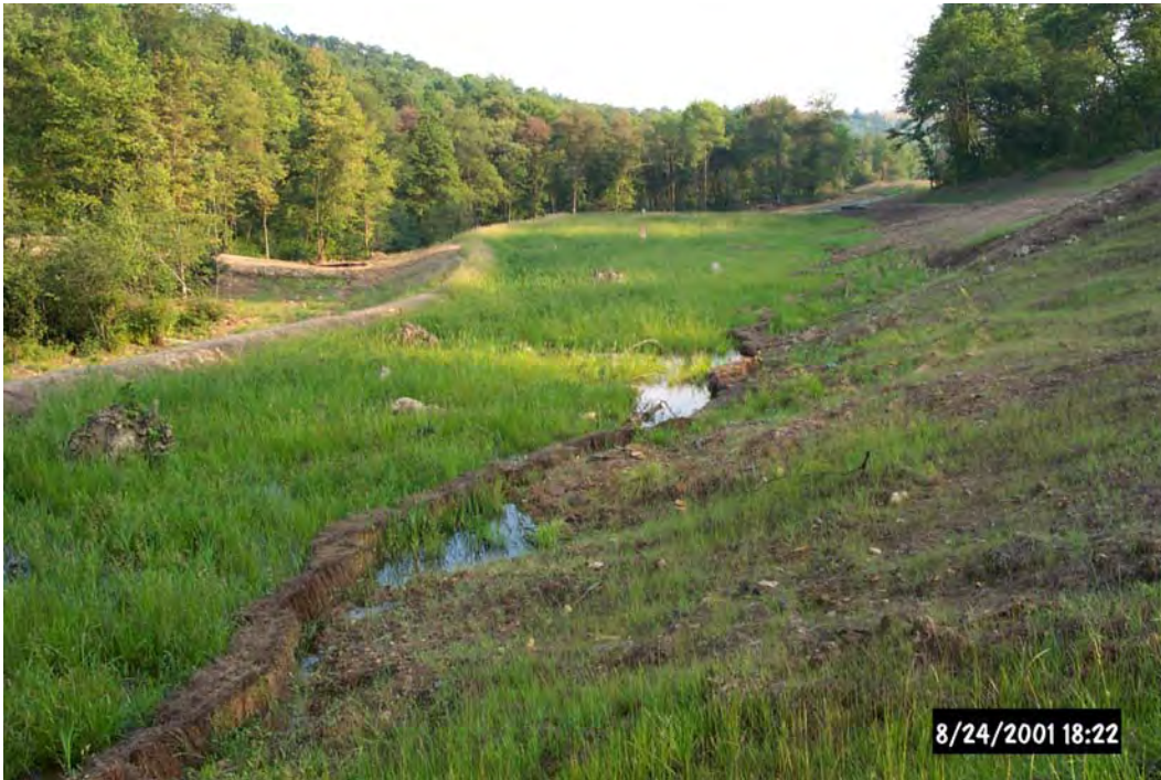
Final polishing wetland, the final component of the passive treatment system, in August 2001 only 1 month after planting by volunteers.
