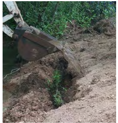
Installation of willow wattles in riparian area (south of stream crossing). (8/8/01)
