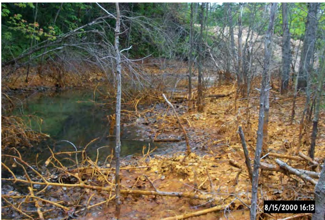
Pre-construction: the ST39 discharge flows into an abandoned strip pit from an old underground mine.
