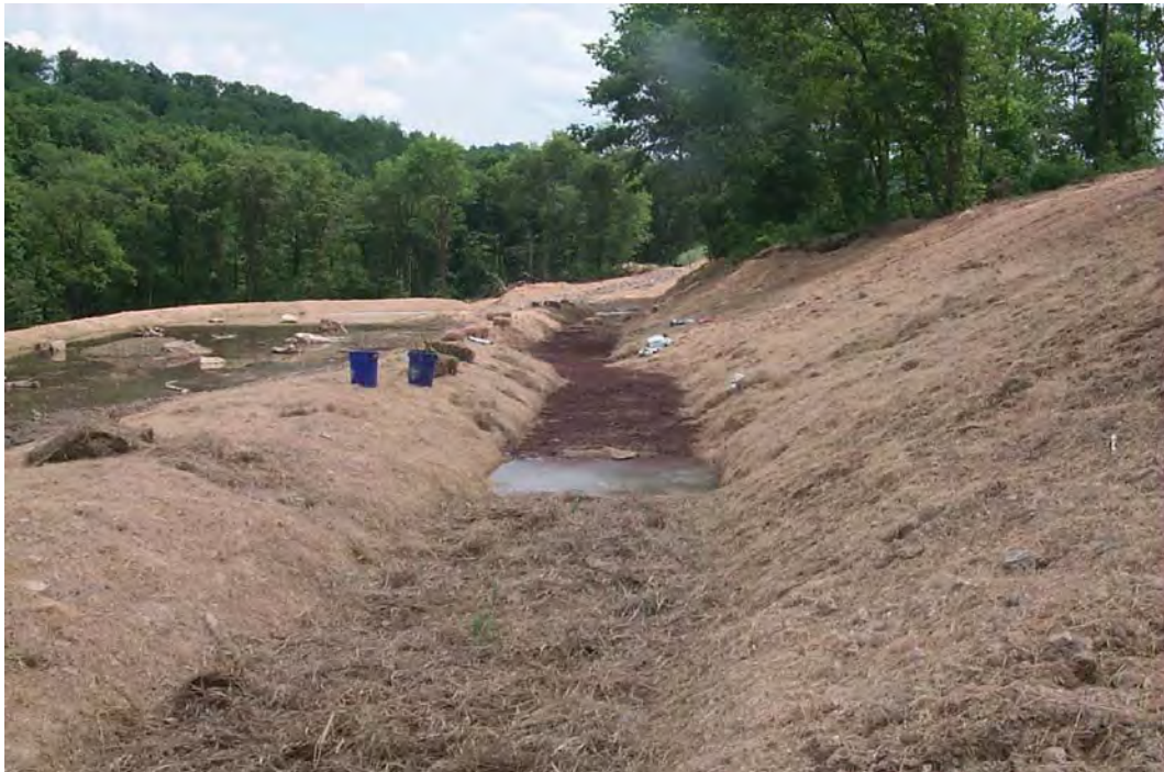
Initial soil amendments, seeding and mulching of Bioswale. (6/20/01)
