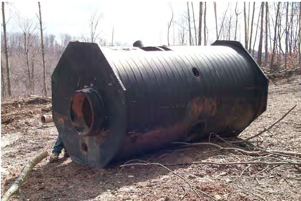
HDPE Manhole used as artificial cave for bat hibernaculum. (3/23/01)
