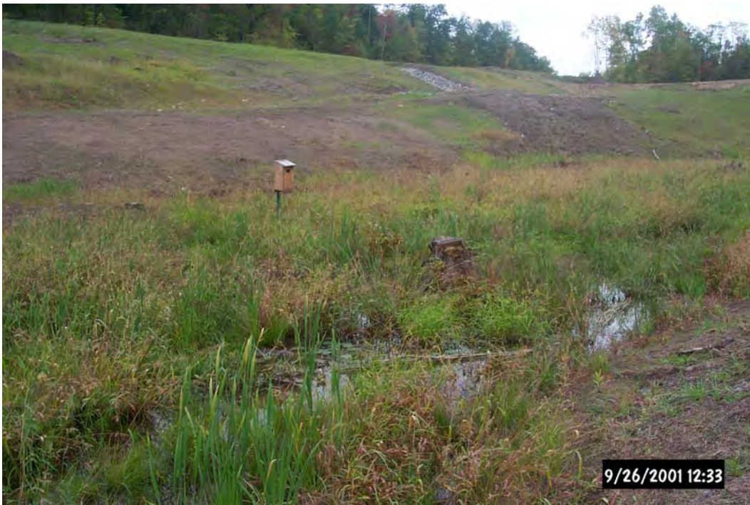
Final polishing wetland two months after planting. Effluent from this final component discharges into Murrin Run.
