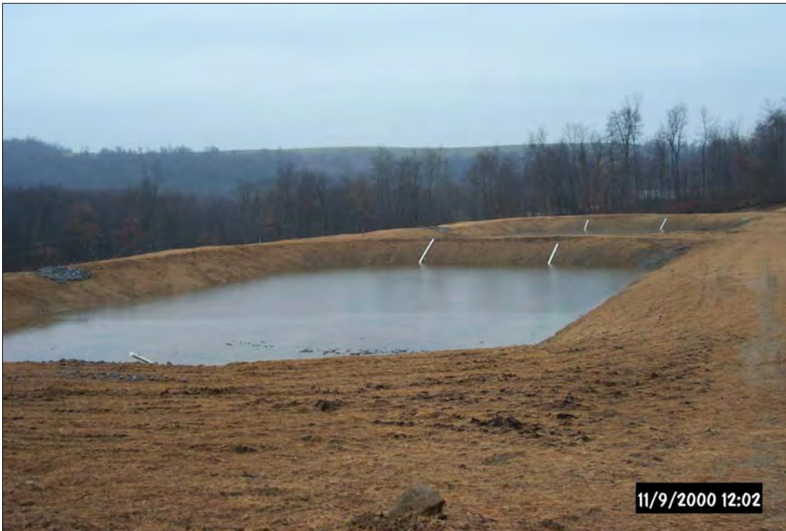
Vertical Flow Ponds #1 and #2
