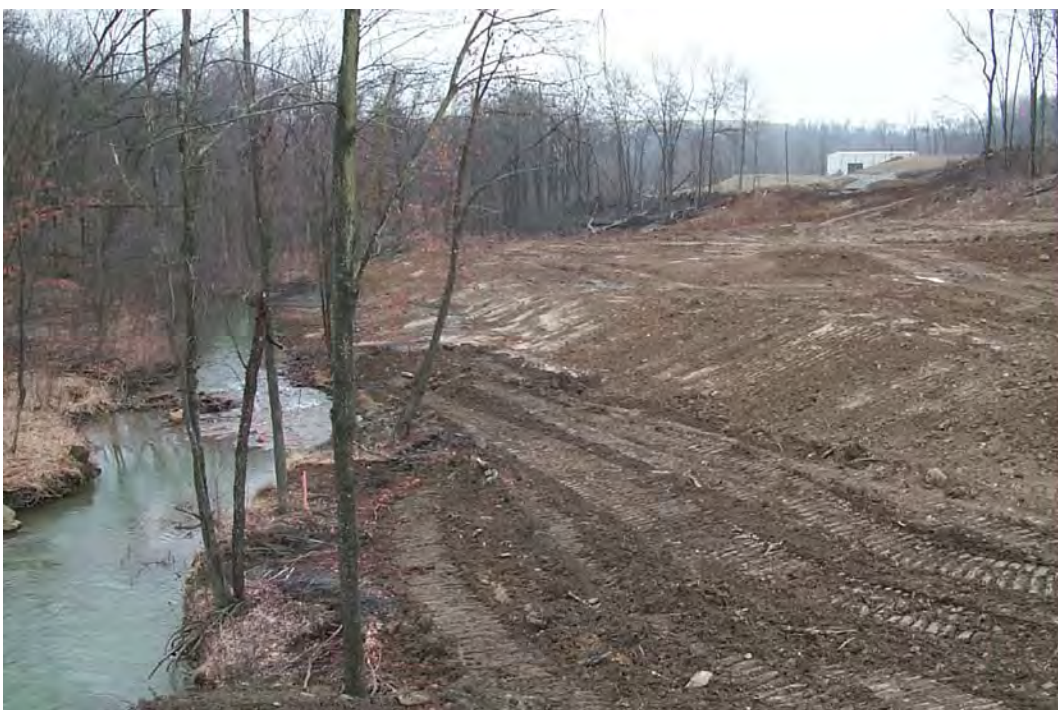
Riparian area (south of stream crossing) with addition of topsoil. (4/4/01)
