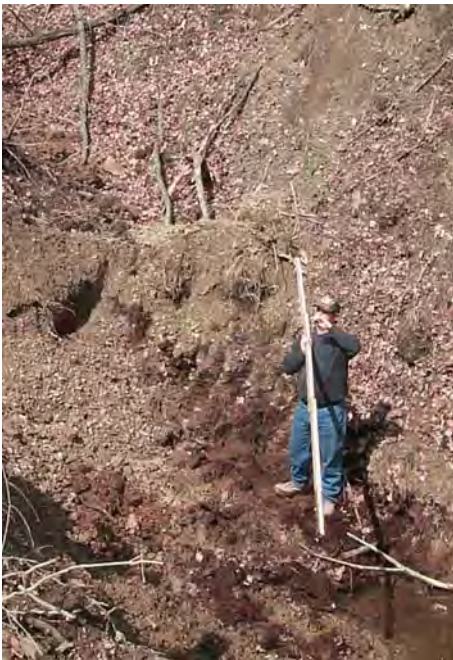
Stadia rod and laser level used to set the hibernaculum and tunnel to appropriate depth and slope. (3/23/01)
