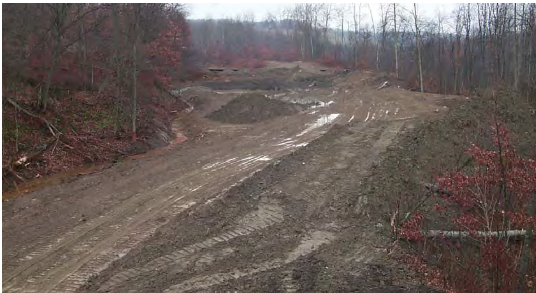
ST41 Upper Wetland under construction. (11/13/00)
