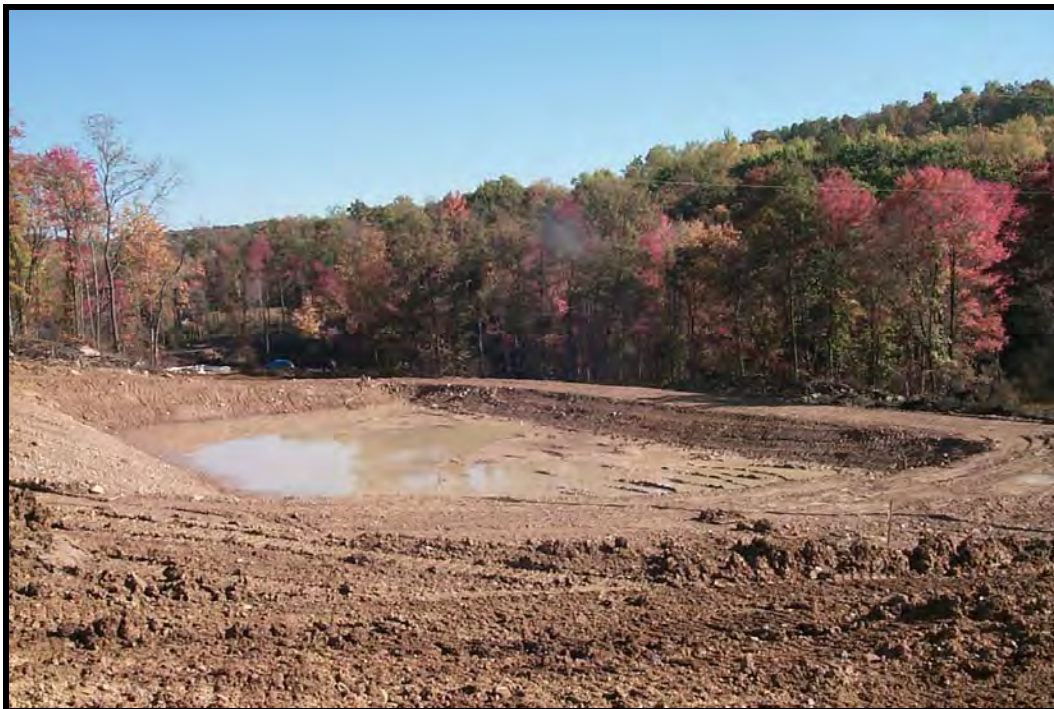
Basin excavated for the ST 38/39 treatment wetland. (10/12/00)
