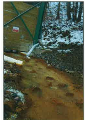
Concrete lined channels convey the water to and from the dosing system. Rocks were anchored into the effluent channel to assist in mixing the hydrated lime. The site lacked adequate fall between the doser and settling basin to promote mixing.
