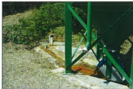
Concrete lined channels convey the water to and from the dosing system. Rocks were anchored into the effluent channel to assist in mixing the hydrated lime. The site lacked adequate fall between the doser and settling basin to promote mixing.
