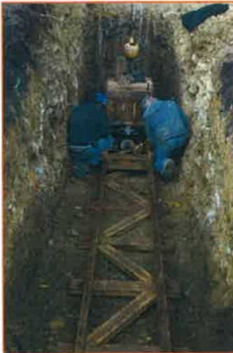
Winters Contracting then bored through the coal until they intercepted the mine entry.
