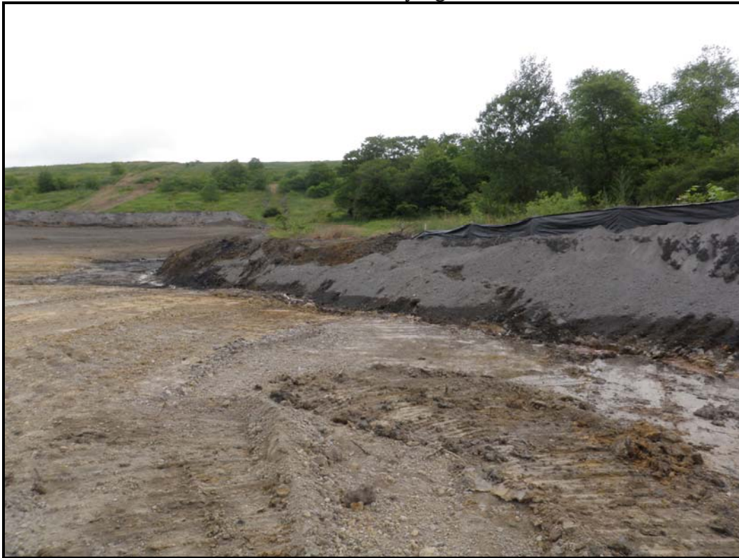
6/14/11 – Mineral CSA Overlying NFG Coal Refuse
