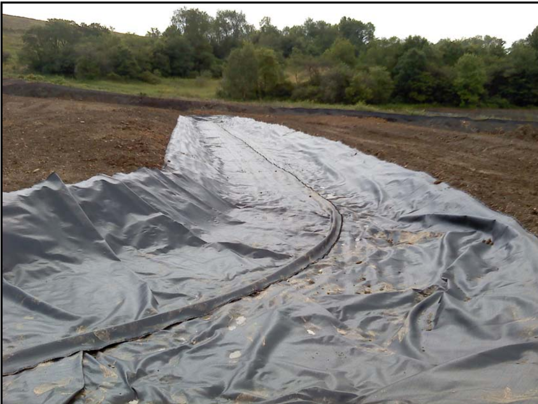
7/19/11 – OPC Installation of Geotextile Liner
