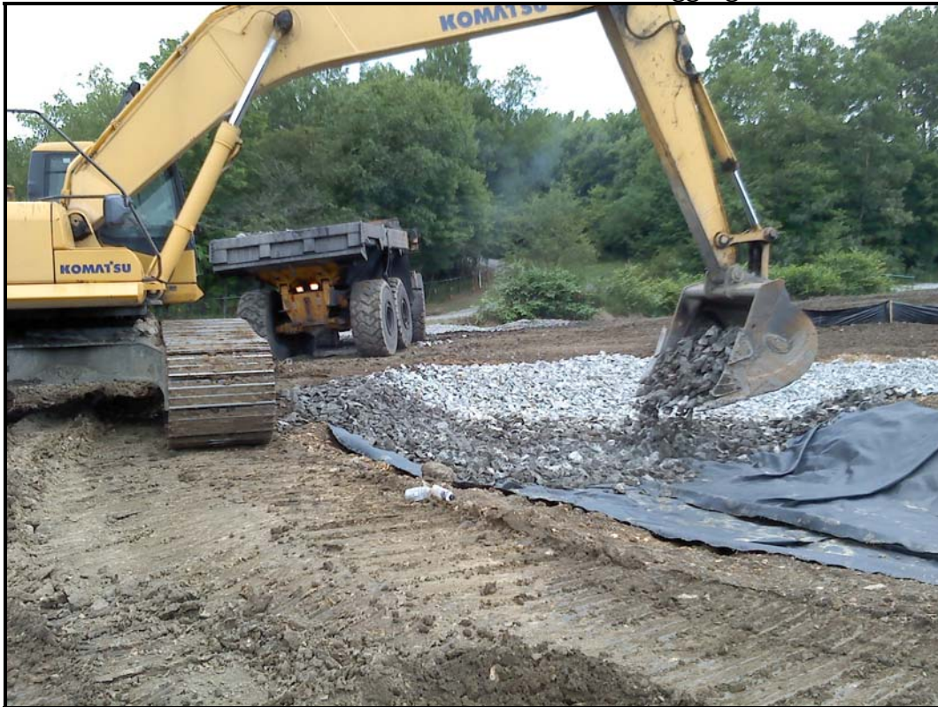
7/19/11 – OPC Placement of Limestone Aggregate
