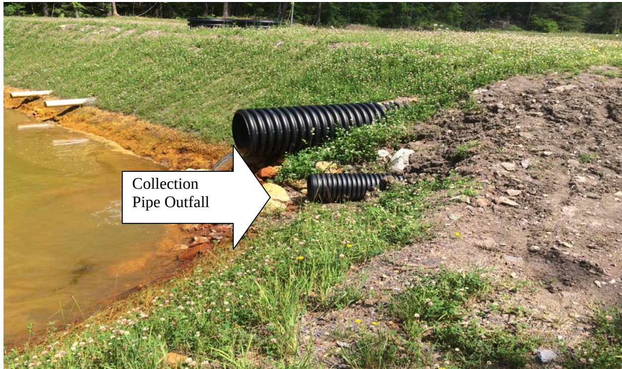
Photo 10: Collection Pipe Outfall at SBD (Prior to Seeding)
