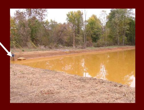
The pond shown after collecting water from the drilling process. The purpose of the pond was to gather water and allow iron oxide the opportunity to settle prior to water entering the Loyalhanna Creek.
