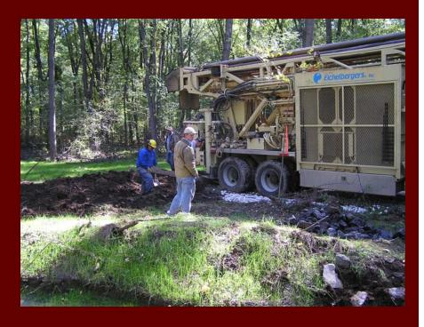
Part II – Hole #1 being drilled by Eichelberger Drilling on October 6<sup>th</sup>. The drill rig moved 175 feet down without encountering a mine void or artesian flow.
