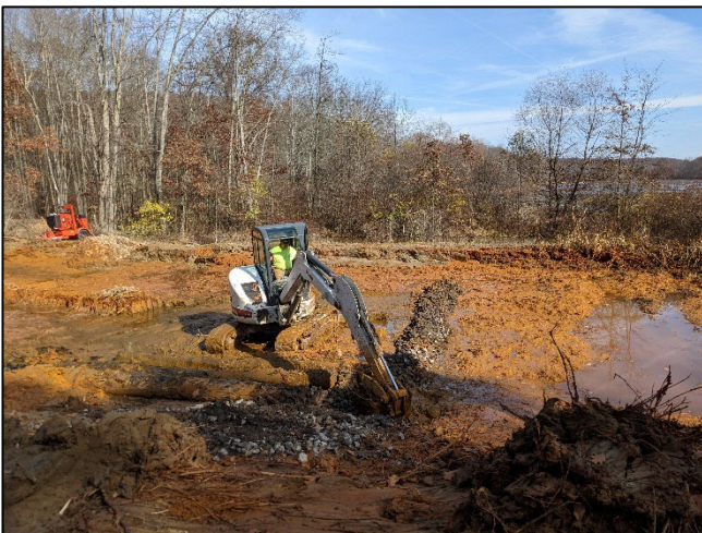
Placement of Level Spreader in Wetland
