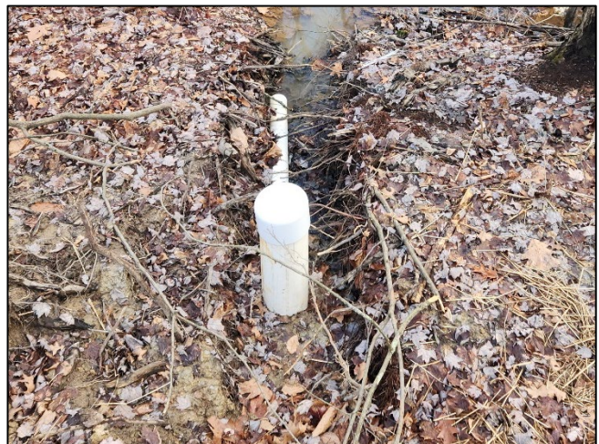
Dewatering Valve in Riser with Cap
