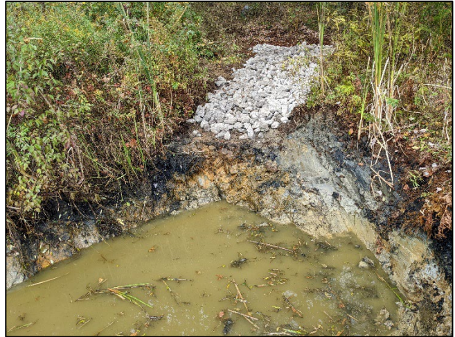
Construction of Spillway for Wet Zone to Collection Pond
