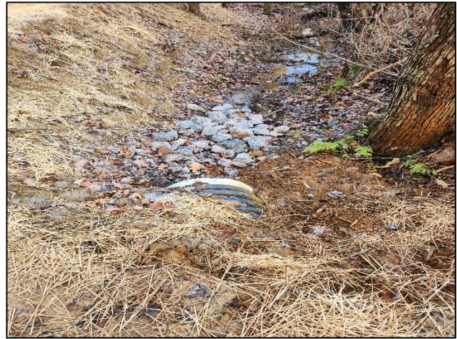
Rock Lined Outlet of 24" N12 Culvert Pipe
