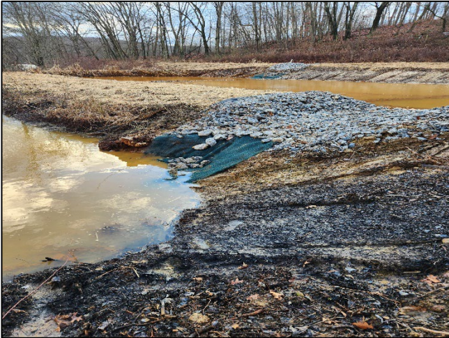
Turf Reinforcement Mats at Outlets of Spillways
