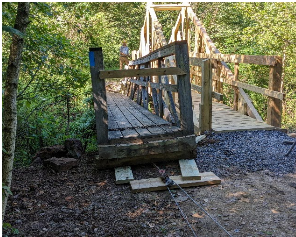
Removing old bridge.
