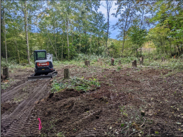
Clearing and Grubbing
