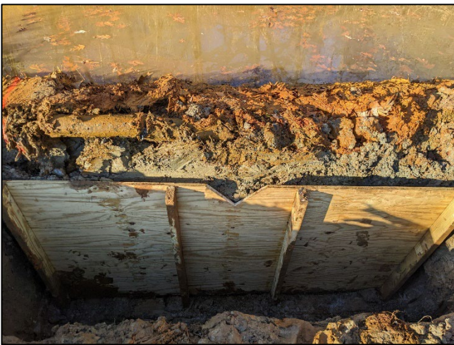
Construction of 6" 90° V-Notch Weir
