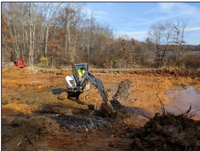
Sludge Removal From Wetland
