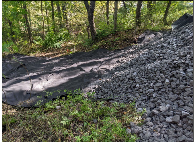
Placement of Geotextile for Site Entrance and Placement of AASHTO #1 aggregate
