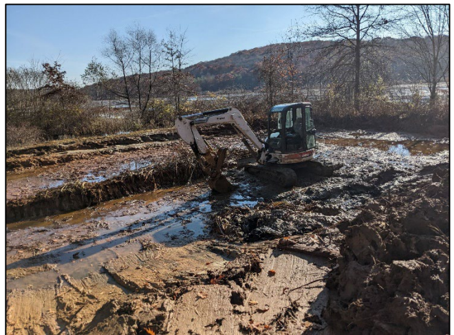
Sludge Removal From Wetland
