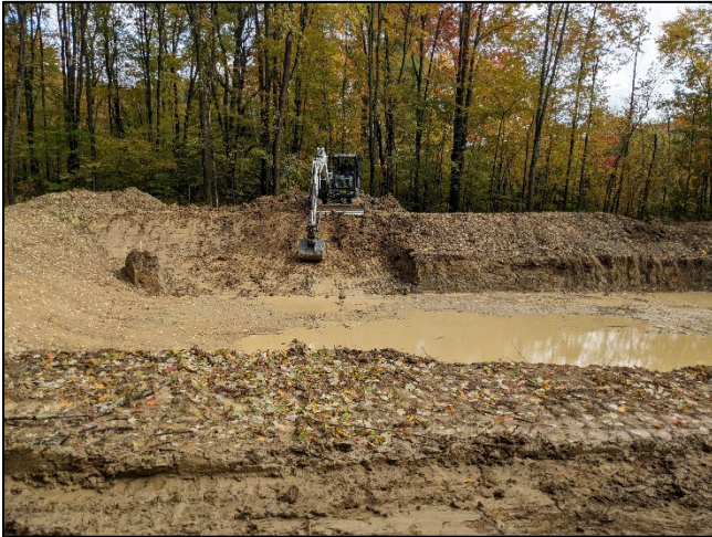
Forming Interior Slopes of Sludge Pond
