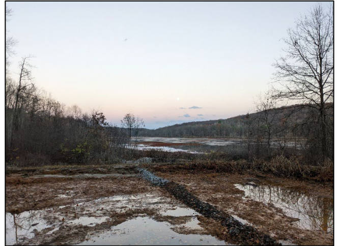
Overview of Level Spreader Across the Width of Wetland
