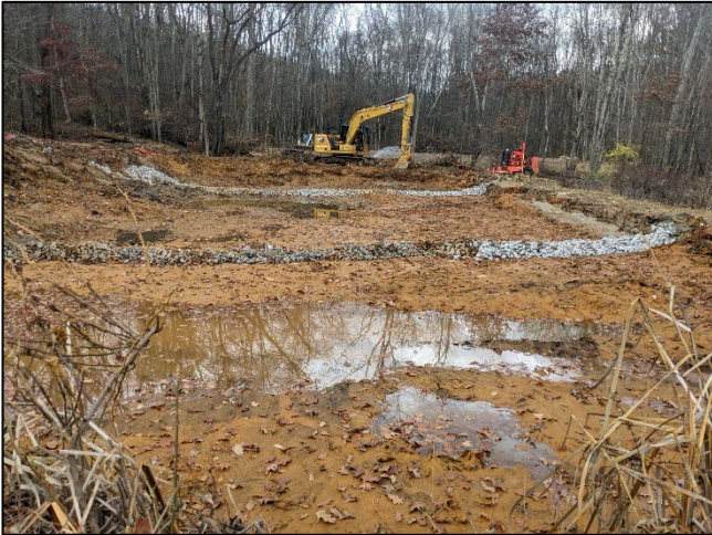
Level Spreaders Across the Width of Wetland
