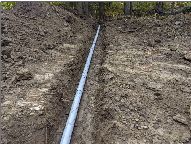
Dewatering SCH40 PVC Outlet Pipe
