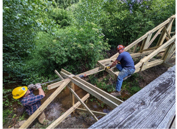
Pulling new bridge across stream.
