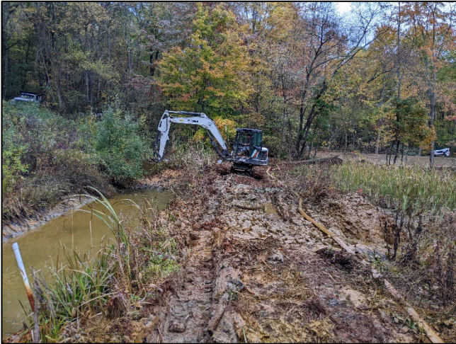
Removal of Sludge and Vegetation from Collection Pond
