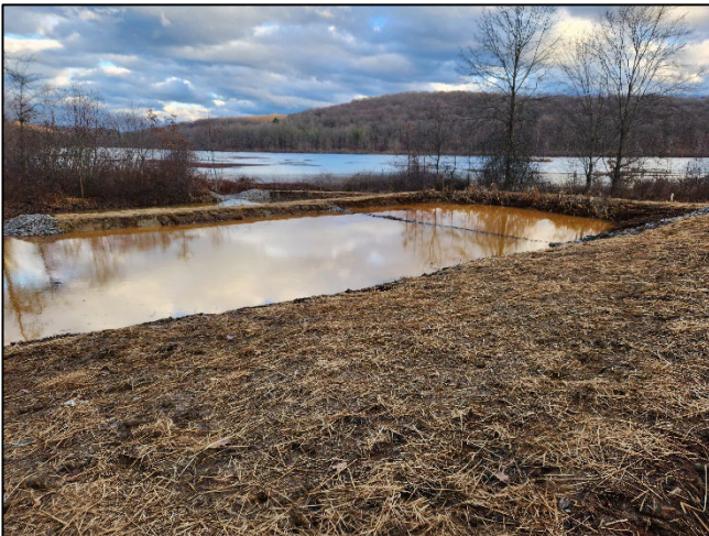
Seeding and Mulching of Wetland Berm
