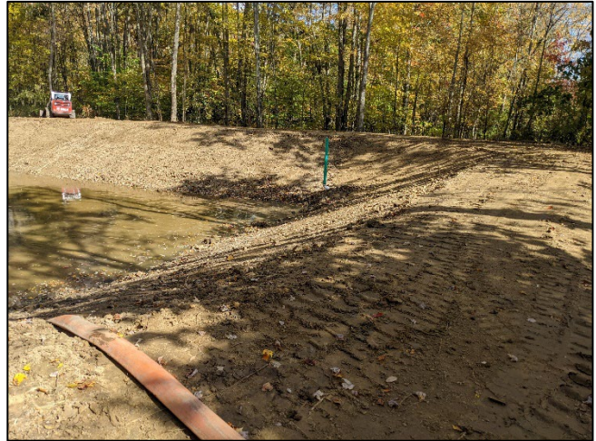
Sludge Line Filling Sludge Pond and Dewatering Riser
