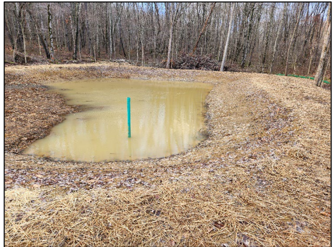
Filled Sludge Pond Post Seeding and Mulching of Sludge Pond Berm
