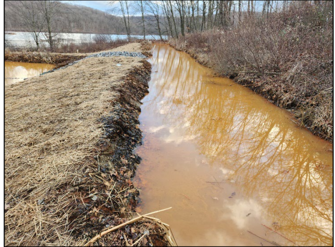
Seeding and Mulching of Collection Pond Berm
