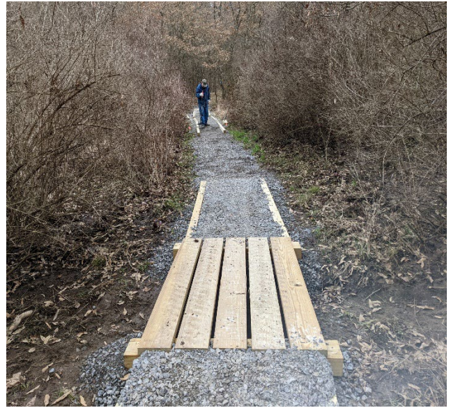
Improved built-up sections with small bridges to allow future flooding to flow across the trail.
