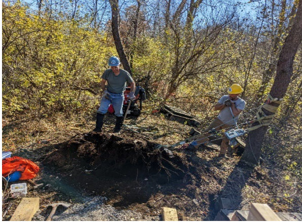
Stump removal with grip hoist.
