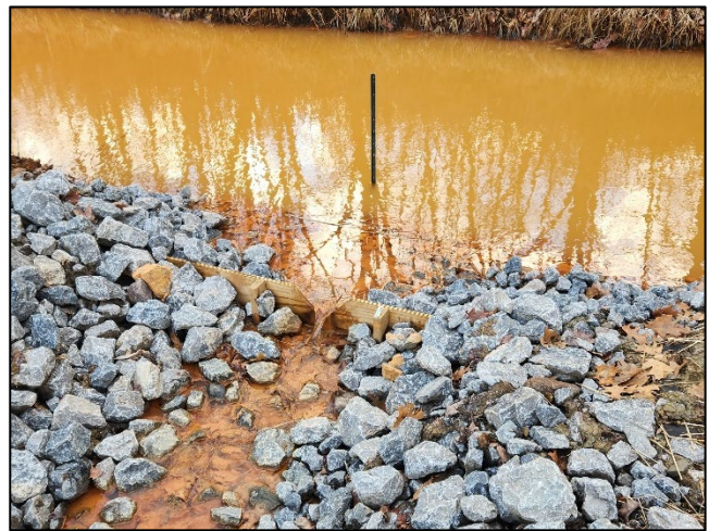
As-Built 6" 90° V-Notch Weir in Spillway
