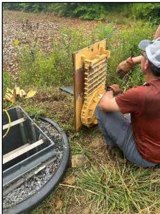
Top Left: Using Jetter to remove iron oxide and other sediments from pipeline to mine seal (6/13/24).
