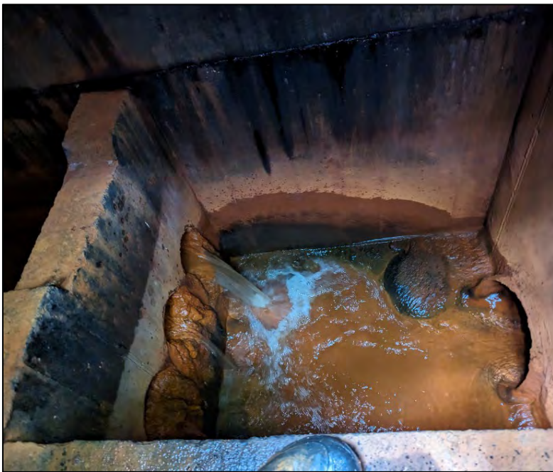
Top Left: Mine Discharge Sample Point 436 improved with an access deck and baffles (8/25/23). Top Right: Pumping water to clear material from forebay outlet pipe (8/25/23). Bottom Left: Iron occluding splitter box components, noted after flow was restored (8/24/23). Bottom Right: Various methods were attempted to clear sediment from the system pipes (8/25/23).
