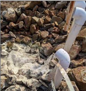
**Top Left**: Wetland flow monitoring pipe was bedded in bentonite (3/1/23).
