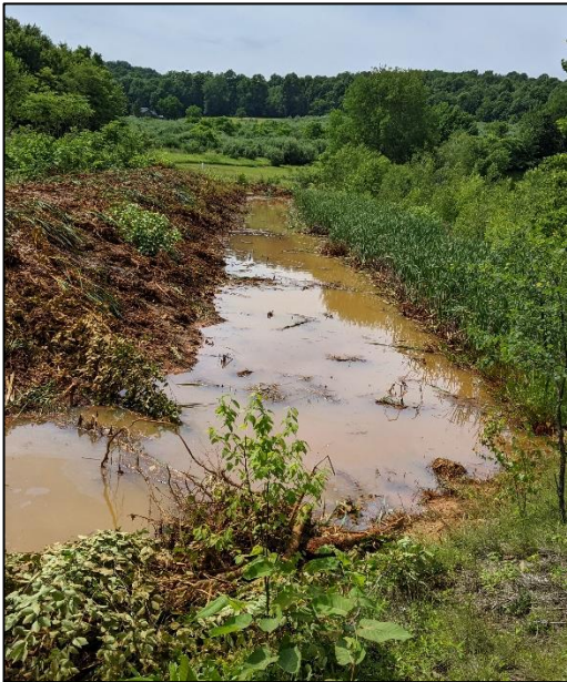
Top Left: Media within the vertical flow ponds was in good condition considering system age (7/8/21). Top Right: Outlet weir was restored to working condition and a staff gauge was installed (7/13/21). Bottom Left: Each wetland component was cleared to increase settling capacity and flow (6/25/21). Bottom Right: Large amounts of iron and vegetation were removed from the wetland (6/25/21)
