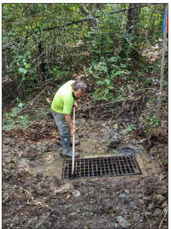
**Top**: BP3-VFW filling with water after stone cleaning and underdrain improvements (8/9/23).
