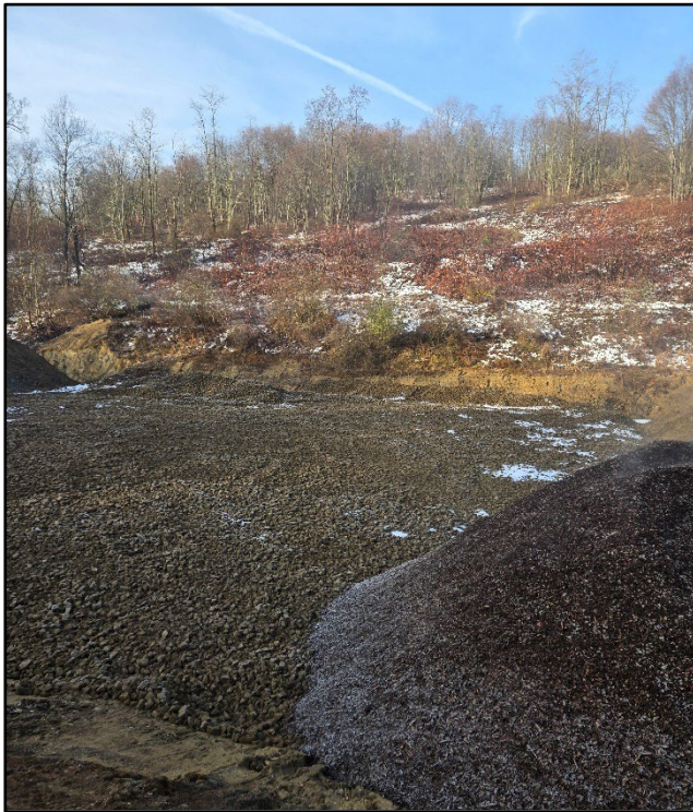
All: Mixing and placement of treatment media in the new JVFPs in November 2024.
