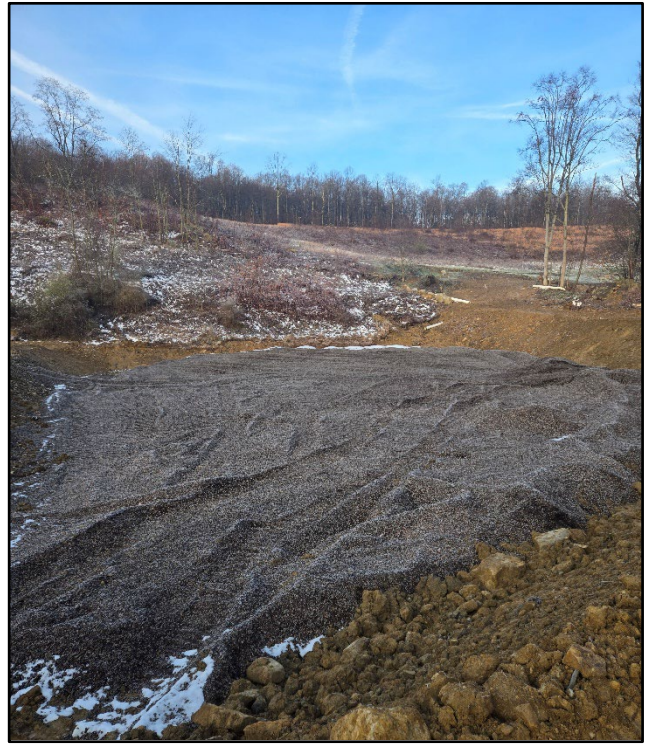
All: Mixing and placement of treatment media in the new JVFPs in November 2024.
