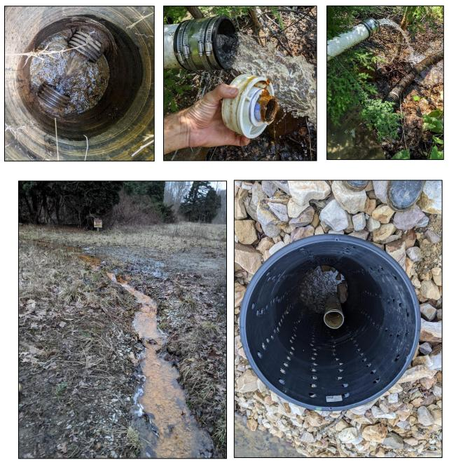
**Top Left**: 2A/2B splitter box has ongoing issues with leaves and debris clogging the pipes (7/27/21). **Top Center:** 2B Bioreactor inlet pipe was cleaned to maintain functionality (7/27/21). **Top Right**: 2B Flow reducer re-installed (7/27/21).
