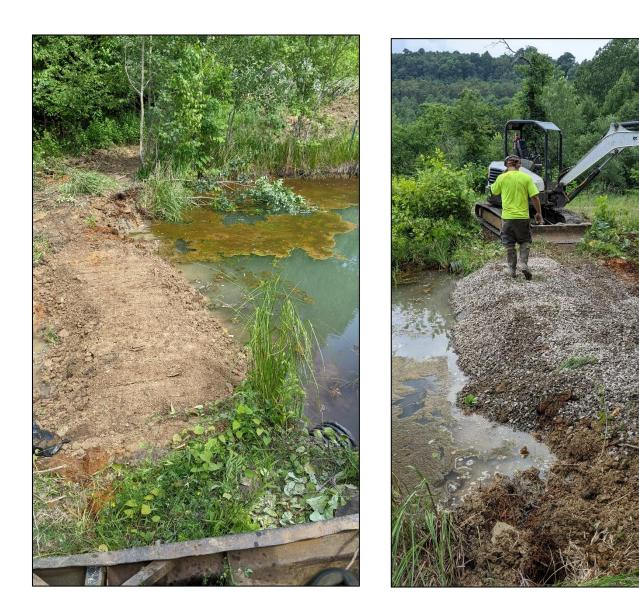
**Left:** The forebay emergency spillway elevation was raised (7/16/21). **Bottom Right:** Geotextile and stone was placed on the new emergency spillway grade (7/16/21).
