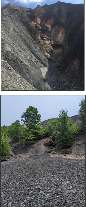
The Tide Coal Refuse pile sits above the Yellow Creek 2C passive treatment system. Channels and ponds had been previously constructed to contain the coal refuse that is eroded during storm events. The BCWA is concerned about the material overtopping and filling in part of the treatment system, which had happened in the past (upper pictures 2/28/19 lower pictures 6/18/21).
