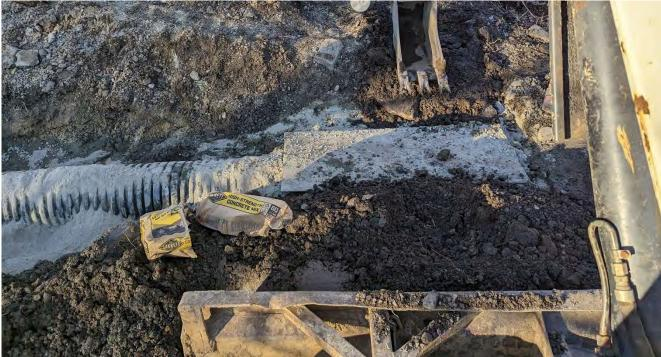
**Top:** A new section of 12" N-12 culvert was installed to replace the damaged sections (3/15/23). **Bottom:** The culvert was bedded in concrete and steel plates were installed above the pipes along the tire tracks (3/15/23).
