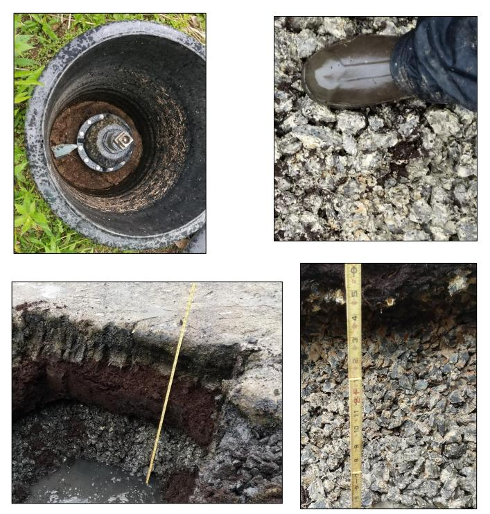
Top Left: 10" PVC valve requires valve tool to open (standard 2" handle).
