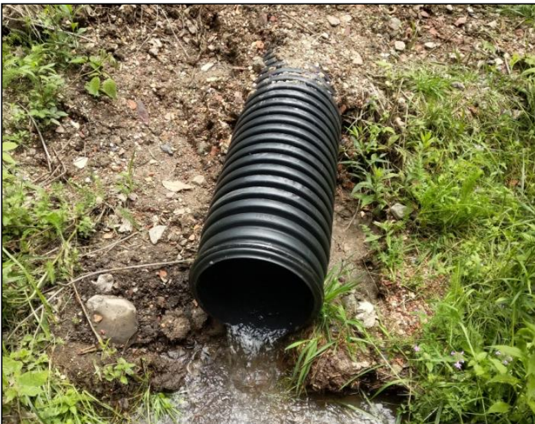
Top Left: ALD clogging led to short circuiting and flow on the access road. Top Right: Limestone in the ALD was generally clean beyond the second monitoring well. Bottom Left: A culvert was installed beneath the access road to act as a temporary overflow (bypass). Bottom Right: A raw water infiltration structure was built as a temporary inlet to the ALD until system redesign.
