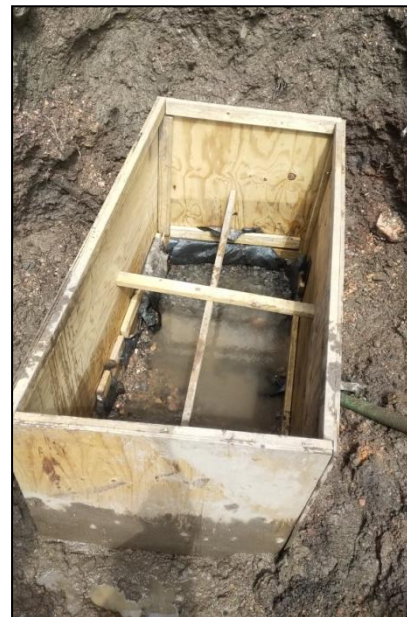
Top Left: ALD clogging led to short circuiting and flow on the access road. Top Right: Limestone in the ALD was generally clean beyond the second monitoring well. Bottom Left: A culvert was installed beneath the access road to act as a temporary overflow (bypass). Bottom Right: A raw water infiltration structure was built as a temporary inlet to the ALD until system redesign.
