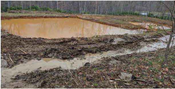
**Top**: HFLB limestone was washed and the outlet pipe reset and extended (4/10/24). **Bottom**: SP1 (top left) and VFP (top right) cleared of woody vegetation and beaver dams. The upslope diversion ditch (foreground) was cleared of vegetation and cleaned as needed (4/11/24).
