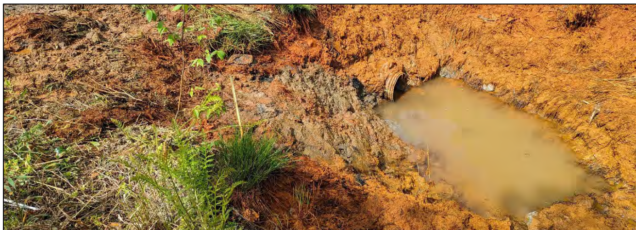
Top Left: Morgan Run 2 bypass pipe from Collection ditch to C-1 clogged (5/16/24). Top Right: Morgan Run 2 bypass pipe from Collection ditch to C-1 was jetted (5/16/24). Bottom: Morgan Run 2 bypass pipe inlet from Collection ditch to C-1 exposed and jetted (5/16/24).
