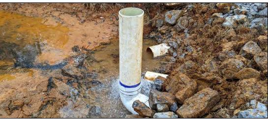
**Top Left**: Test pit in bioreactor shows approximately 0.7 feet of material on top of the media (11/8/23). **Top Right:** Test pit in VFP showing significant accumulation of metals within and above media (11/8/23). **Bottom:** Newly installed secondary VFP outlet riser (11/8/23).
