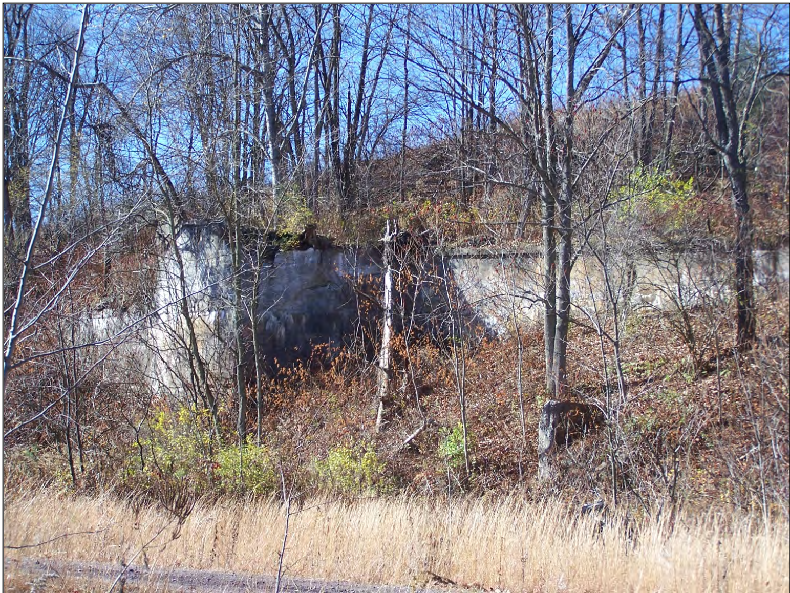
Remnants of the Berwind White Coal Company on the St. Michael Water Treatment Plant site.
