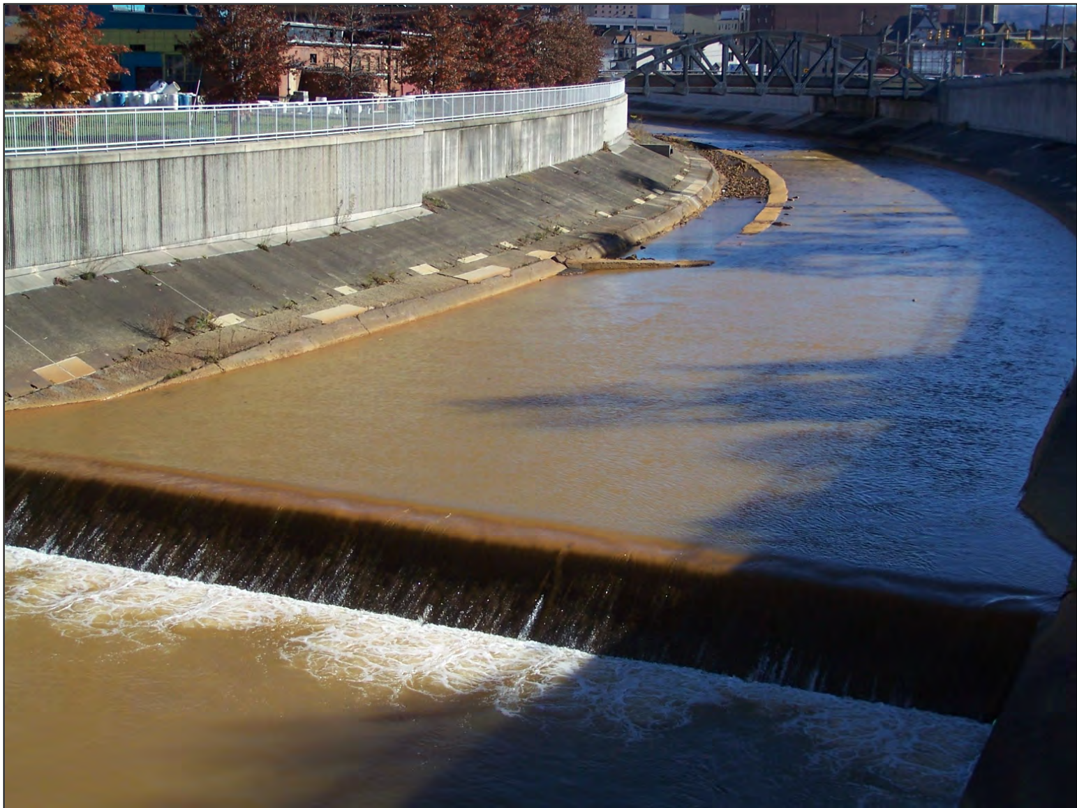
The adverse effect of the AMD on the Little Conemaugh River near the Point in Johnstown, PA. Additionally, Flood Protection Improvement constructed between 1938-1943
