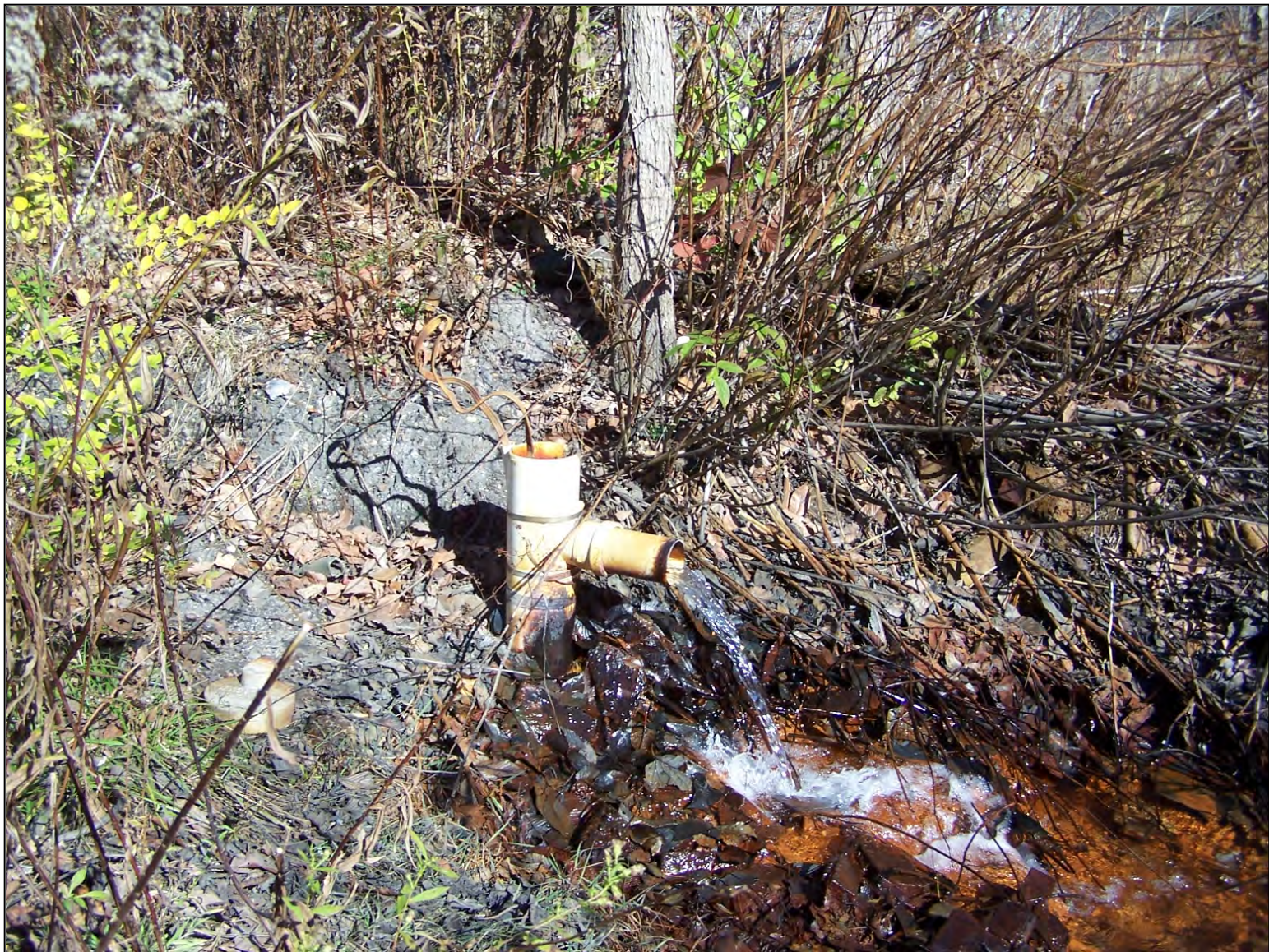
An abandoned well discharging AMD caused by the St. Michael Mine Pool near the shaft. Upon lowering St. Michael Mine Pool residual discharges will cease.
