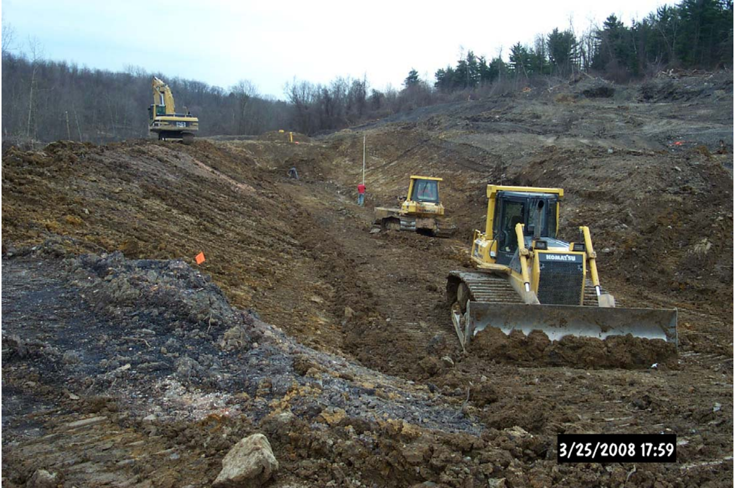
Quality Aggregates Inc. Construction Crew led by site Foreman Wayne Fuchs Building Vertical Flow Pond East (VFPE)
