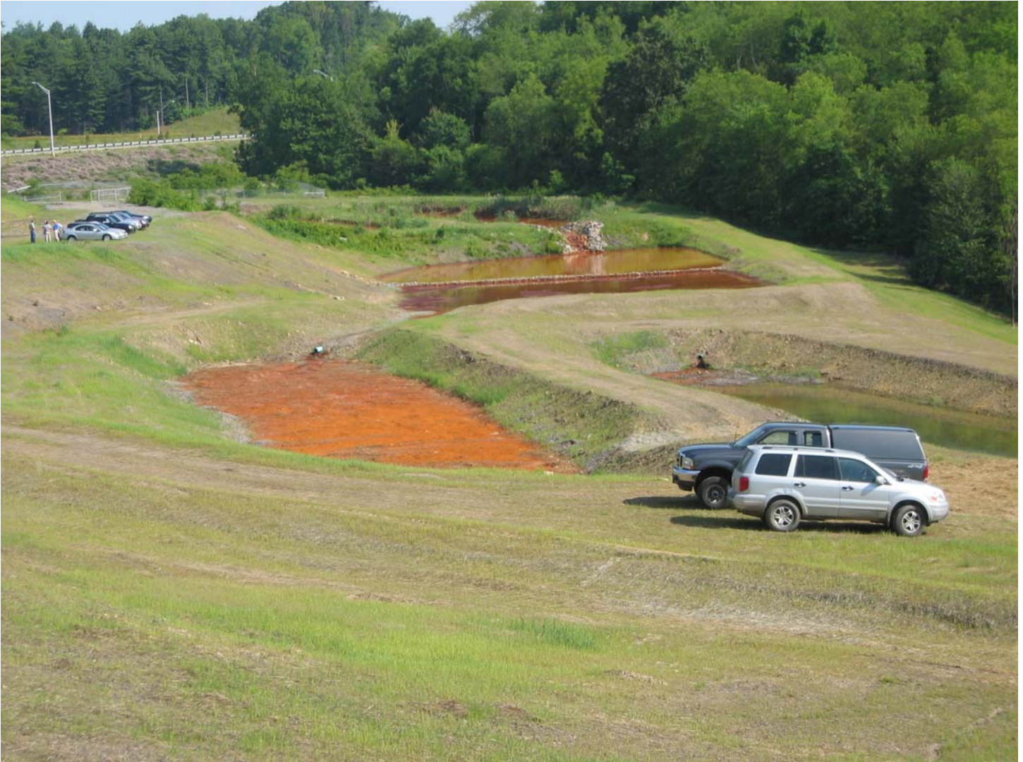
View of the Ponds North Fork Montour facility looking north 06/25/2008. Ponds 1, 2 & 3 in the background and Vertical Flow Ponds (VFPE and VFPW) in the foreground.
