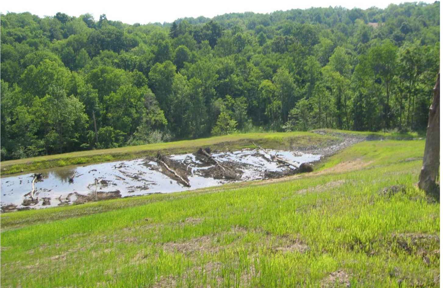
1/3-Acre Treatment Wetland Located at the Bottom of the North Fork Montour Run treatment system (before planting 06/25/2008).
