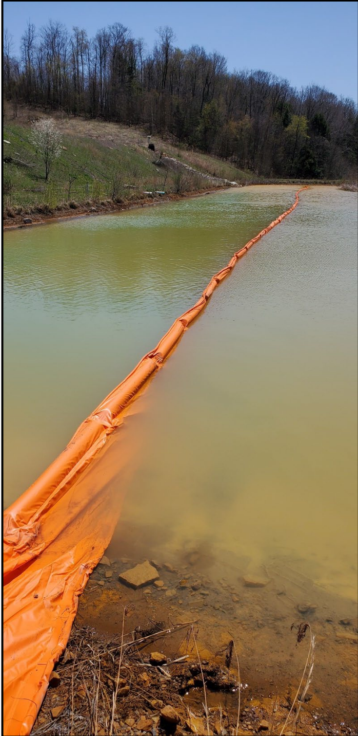
Top: Settling Pond 1 with direction baffle curtain. (9/21/22)
