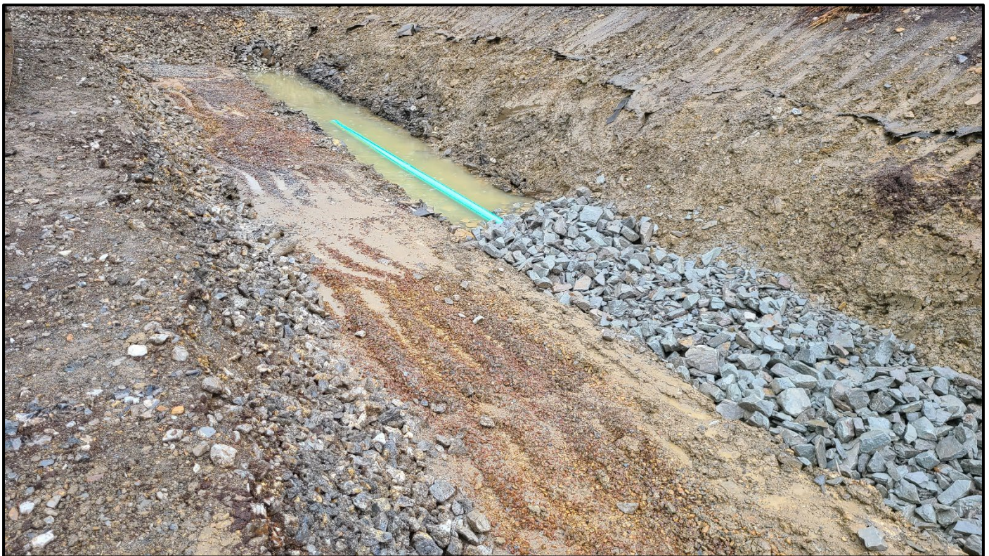
Top: Overview of the dewatering basin. (9/21/22)
