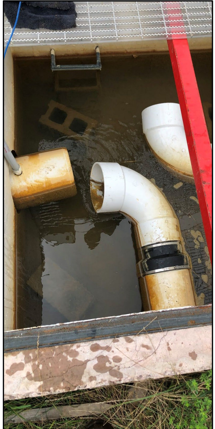
Bottom: Two-Way Splitter with top aluminum grating removed to access 10-inch SCH40 PVC 90° elbows connected to 12-inch SCH40 PVC pipes used to adjust flow to JVFPs. (10/06/22)
