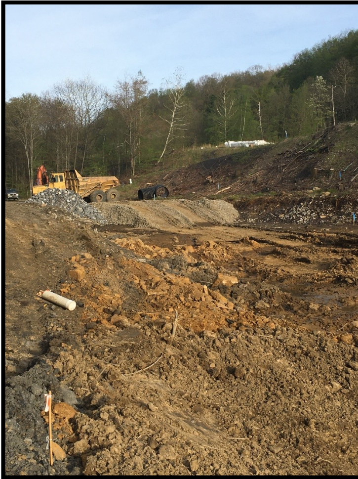
Left: Removing stone in former FeAlMn bed to and excavation of Holding Pond (HP). (5/20/2020)
