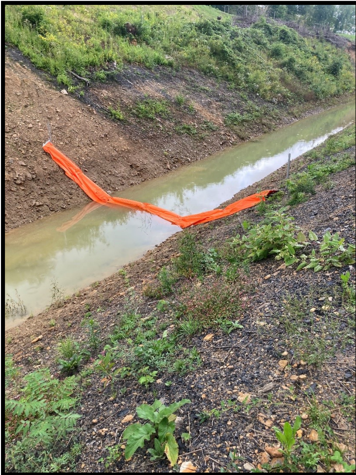
Left: Baffle curtain installed within SP2. (9/10/2020)
