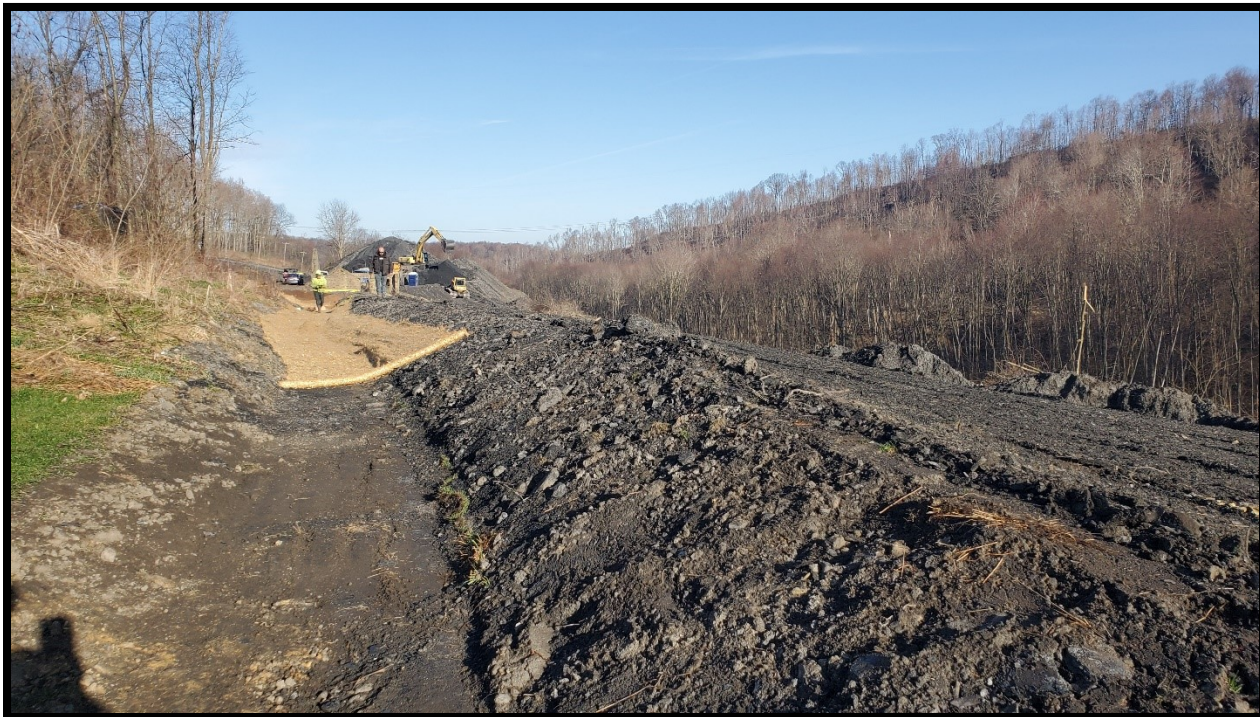
Top: Tree removal preceded construction work. (3/23/2020)
