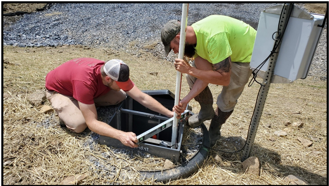
Top: Instillation of the Agri Drain Smart Drain System. (6/25/2020)
