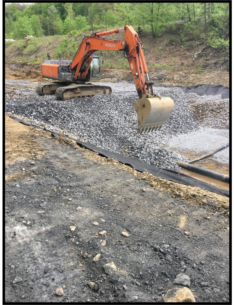
Left: Removing stone in former FeAlMn bed to and excavation of Holding Pond (HP). (5/20/2020)
