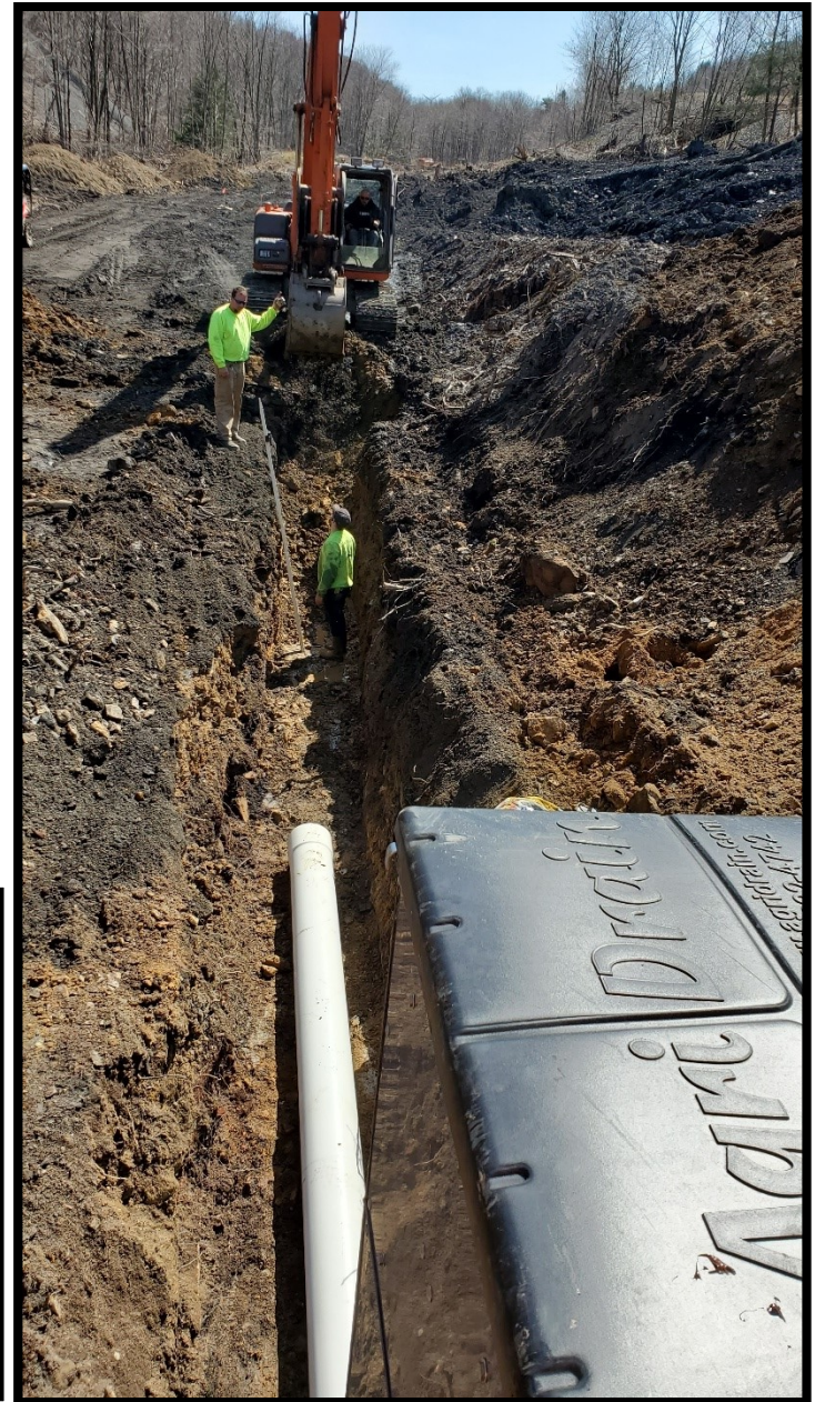
Top Left: Fully excavated Auto Flushing Vertical Flow Pond 2 (AFVFP2) prior to being filled with limestone. (4/29/2020)
