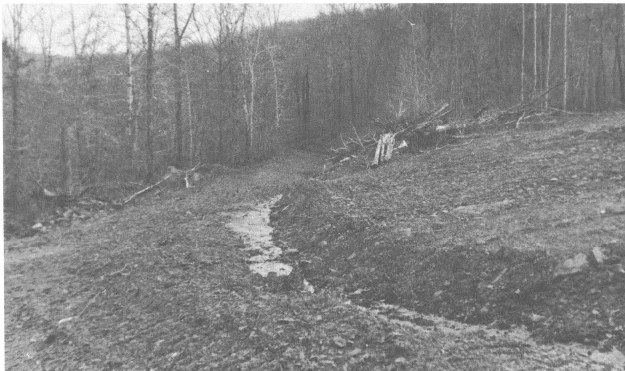
FIGURE 19. - Ditch Constructed to Divert Water Flowing From an Underground Mine in the Northwestern Section.
