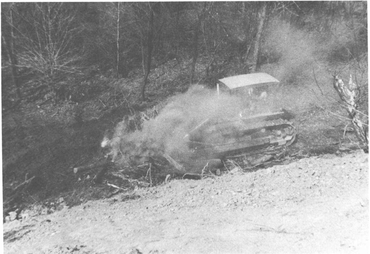
FIGURE 11. - Clearing and Burning Brush and Trees Prior to Site Reclamation.
