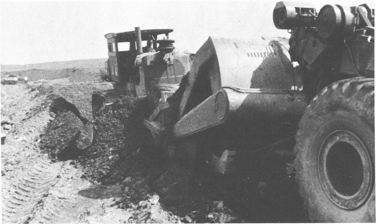
FIGURE 16. - Bulldozer Assisting Scraper in the Northwestern Section.
