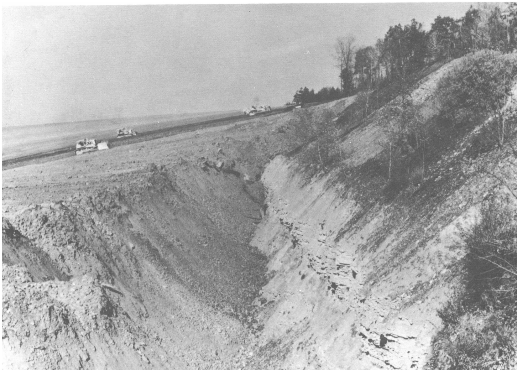
FIGURE 15. - Scene of Reclamation Work Before the Scrapers Were Added to Working Force. Note the distance the material had to be transported.
