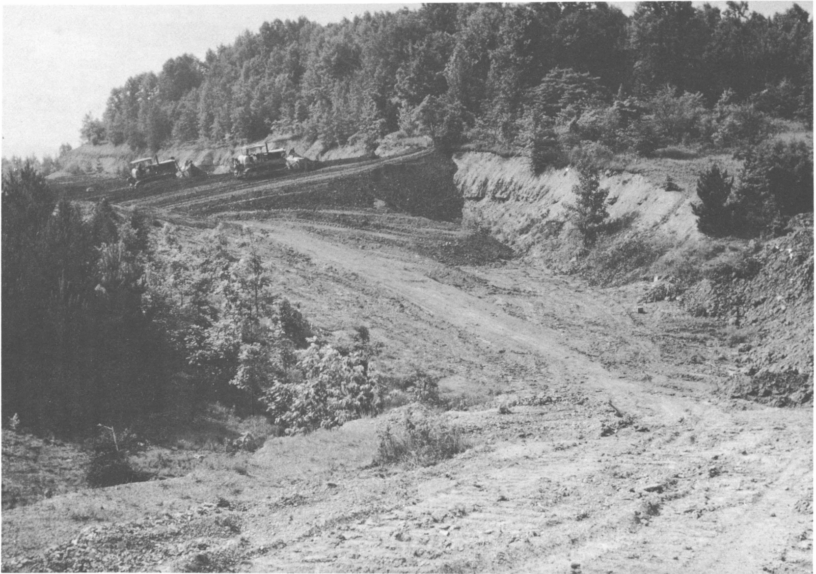
FIGURE 13. - Backfilling of Surface-Mined Area in the North Central Section.
