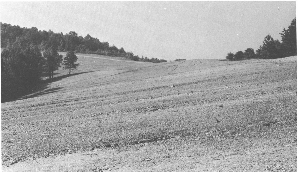
FIGURE 17. - View of Completed Backfilling and Grading in the Northwestern Section.
