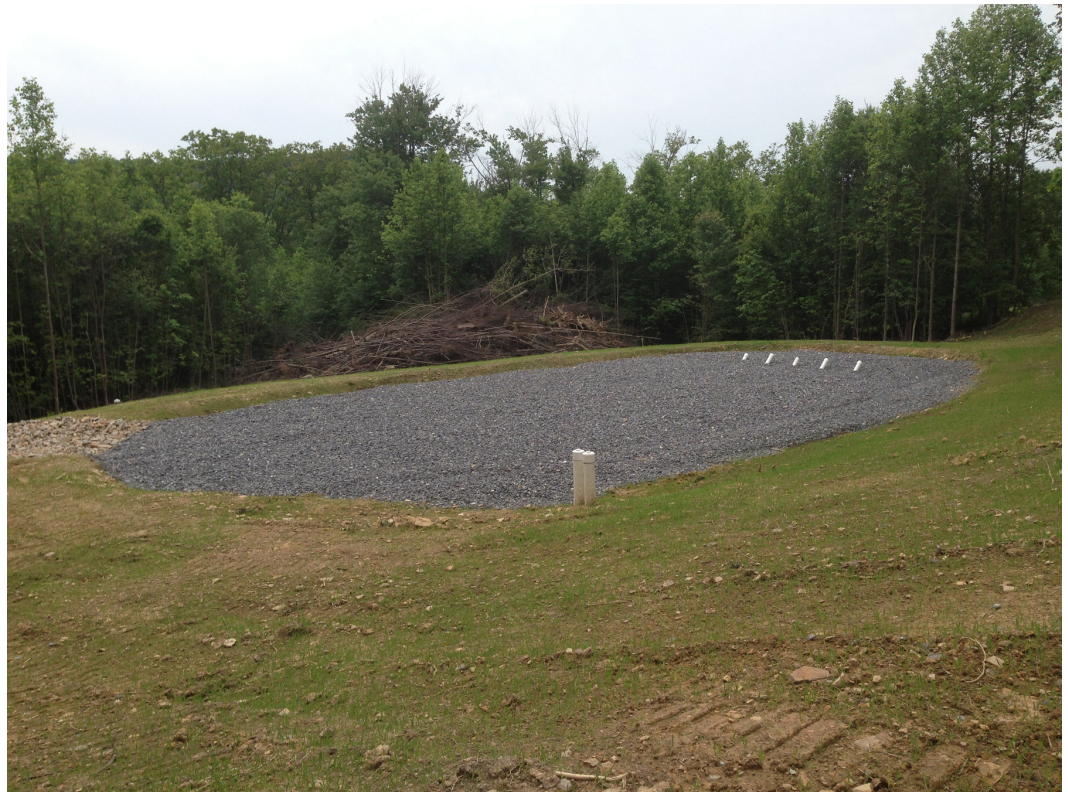
Phase VIII up-flow, manual flush, oxic limestone drain soon after construction.
