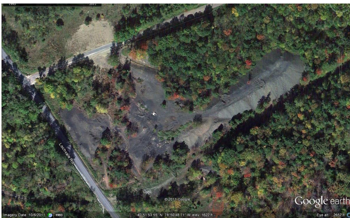
Phase IV site just after mine pool explosion with dual pipe installed and breach reclaimed.
