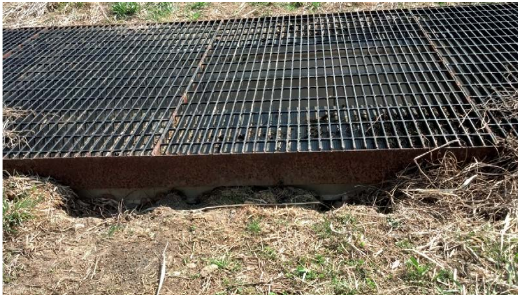
Figure 4. Tripping hazard caused by erosion/animal digging on the sides of the grates.
