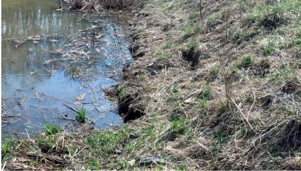
Figure 2. Muskrat damage of a wetland berm.
