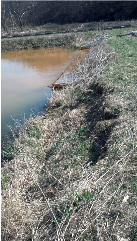
Figure 3. Slumping of the berm between pond 4 and 5 on the pond 5 side.
