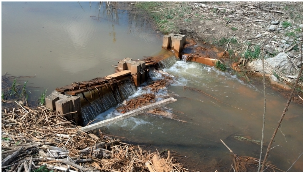
Figure 5. Erosion around the final effluent structure is allowing water to bypass around.
